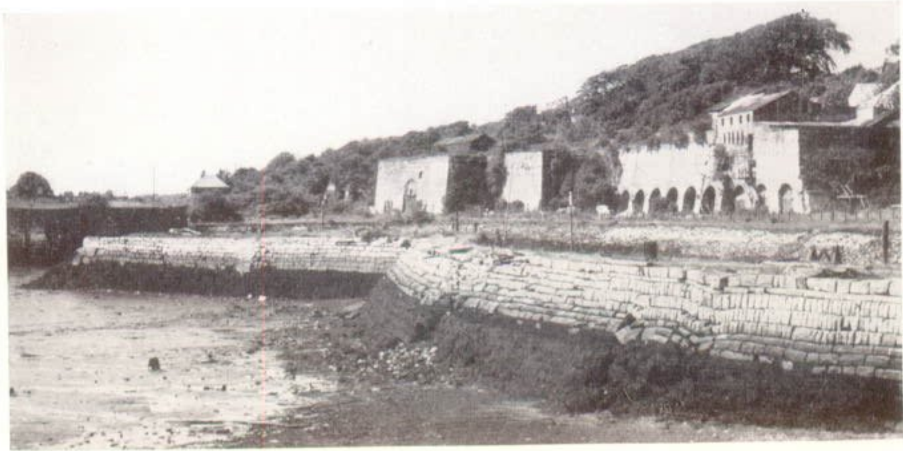
a Charlestown: outside of inner pier from E.
