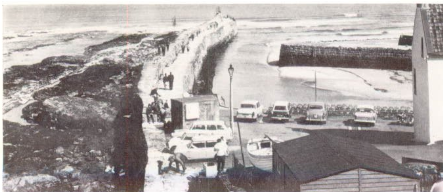
c St Andrews: centre , main pier; right , cross-pier. From W.
