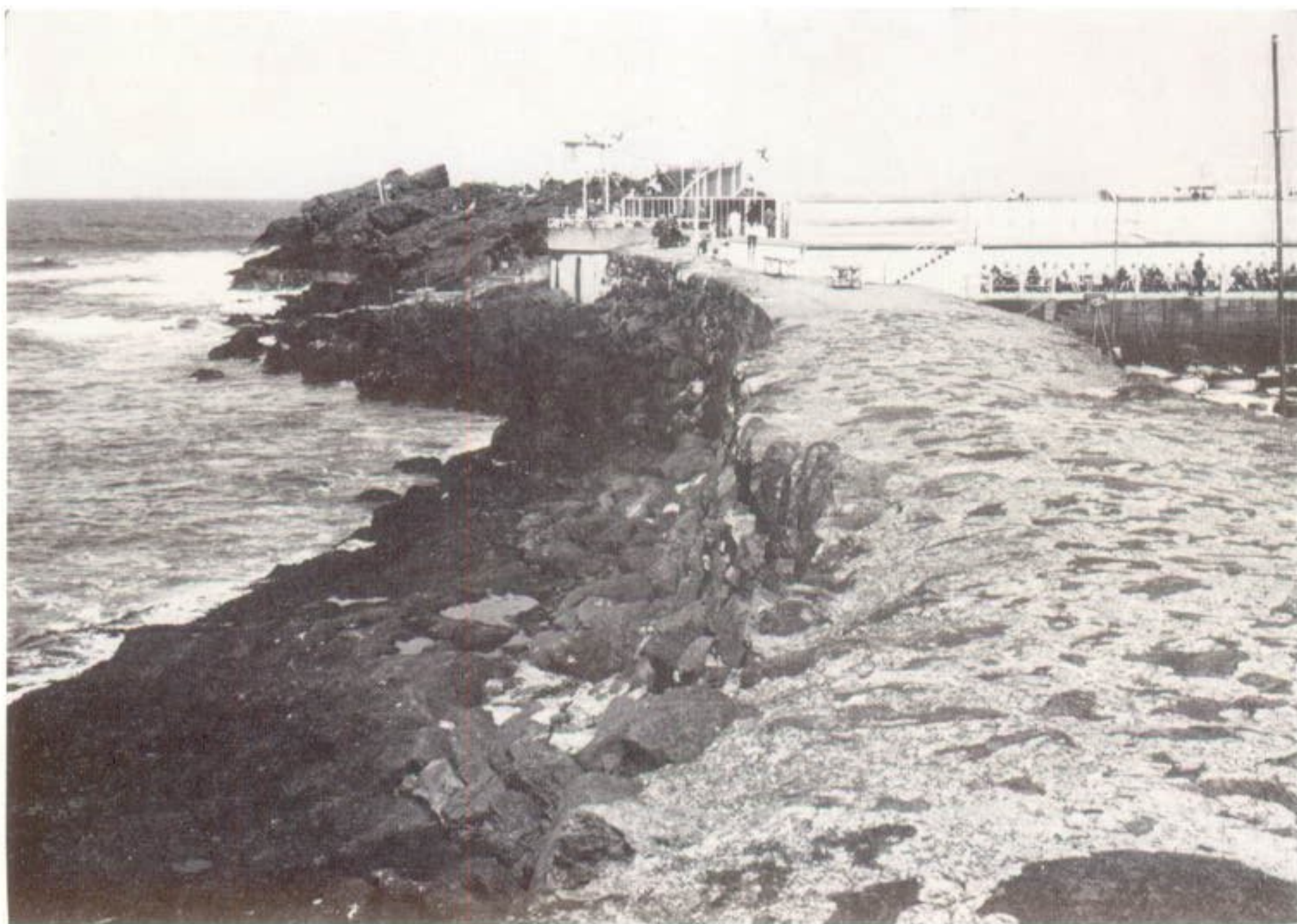
a North Berwick: view NE. along breakwater
