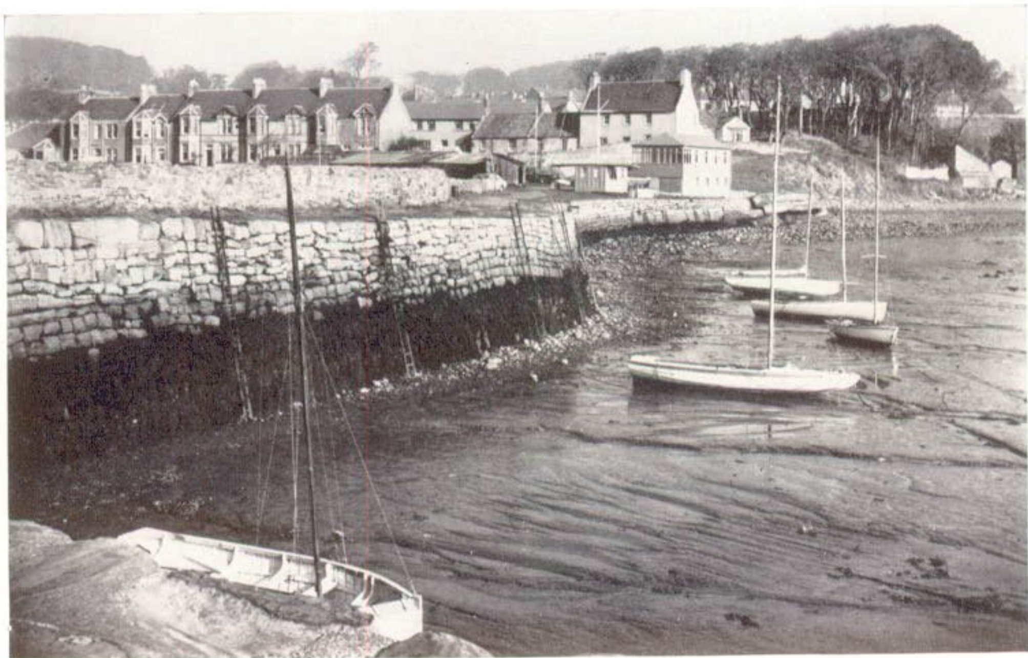
b Brucehaven: pier
