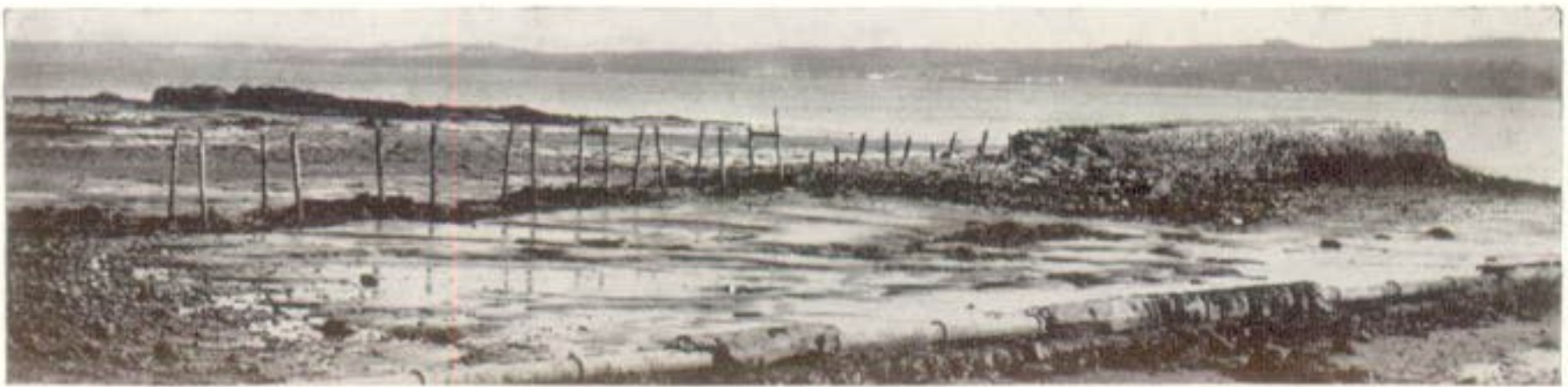
b Culross: pier, from W.
