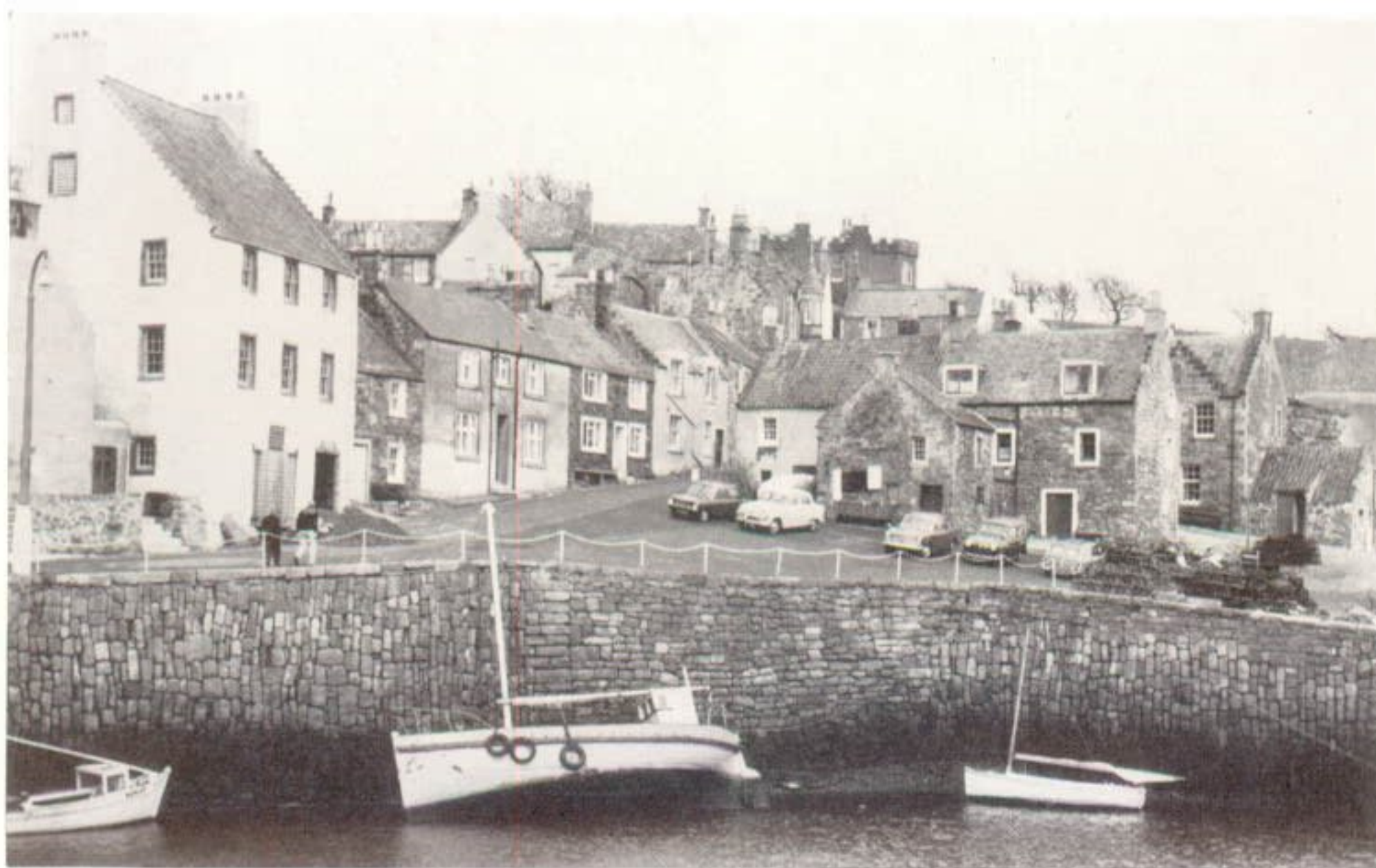
b Crail: N. quay, with vertical masonry and inserted 'patch'
