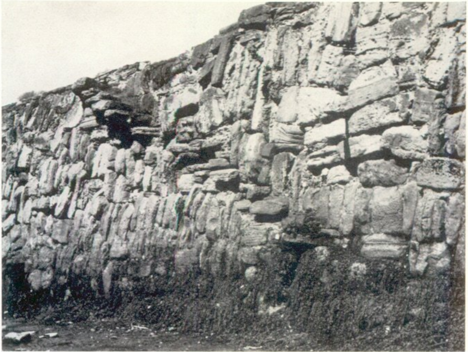
1. Steps on inner face of East Pier
