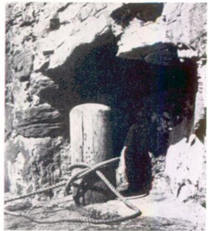
3. Warping-pawl in recess on East Pier
