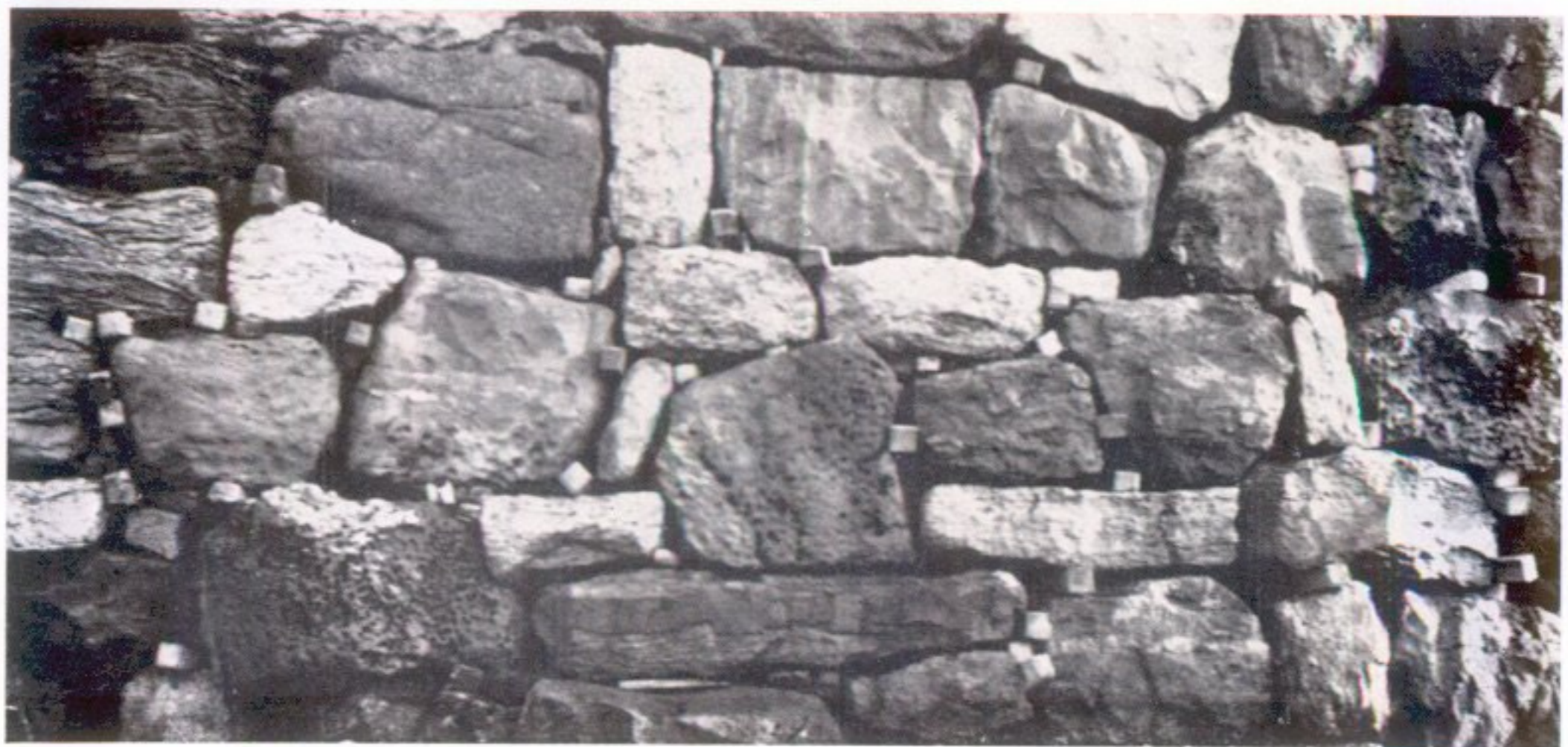
4. Dry-stone breakwater at North Berwick, showing wooden wedges
