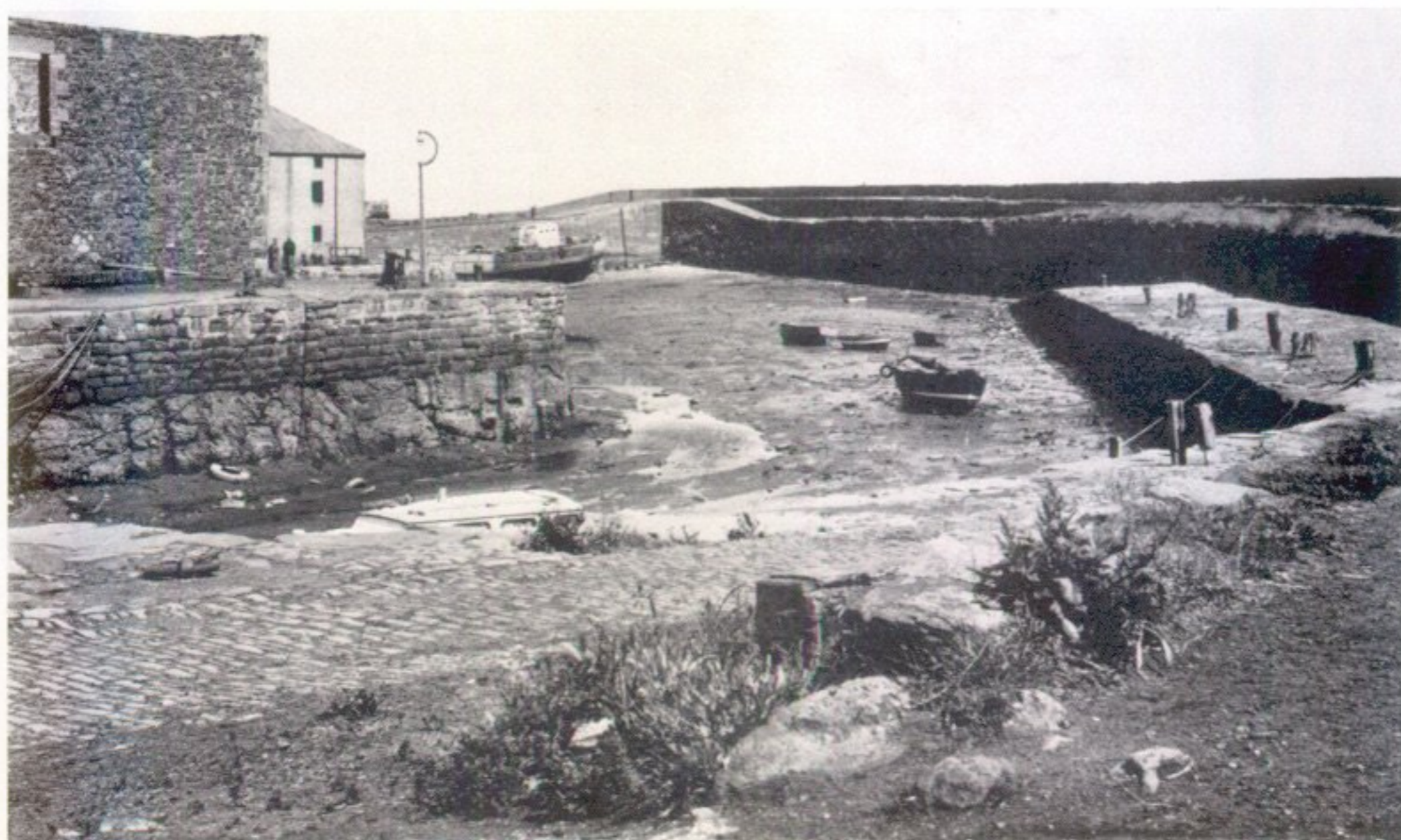
2. General view of harbour from S., showing excavated rock (left) and Coal Wharf (right) with East Pier beyond
