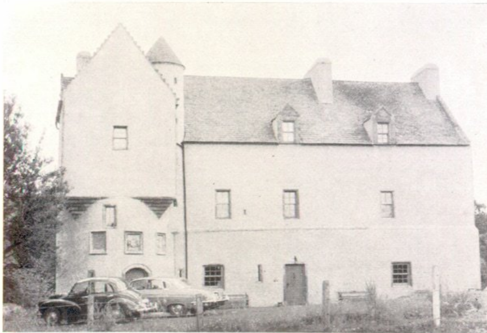
2. North front, general view
