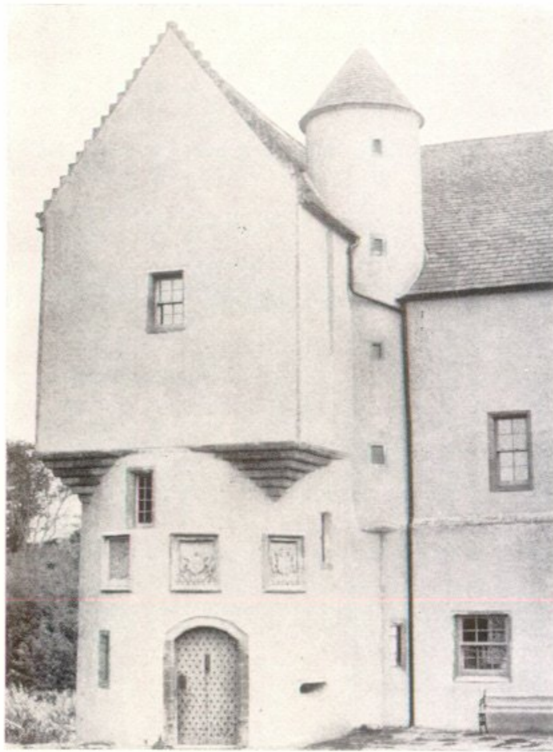
1. North front showing main doorway and stair towers
