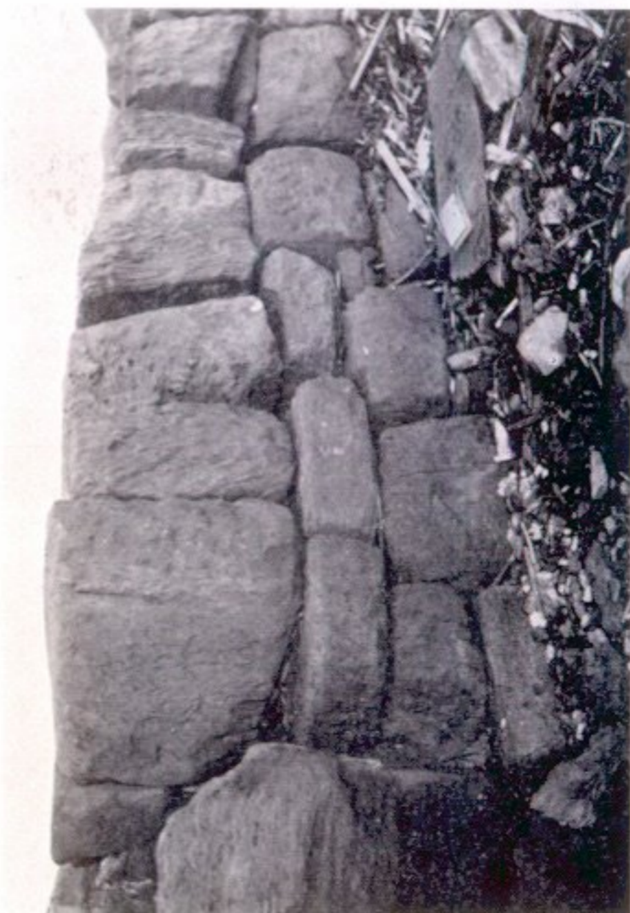
3. Masonry of the inner face of the main pier
