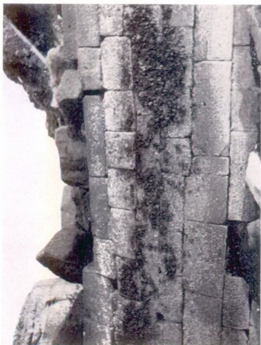
1. Masonry of the outer face of the southern pierhead
