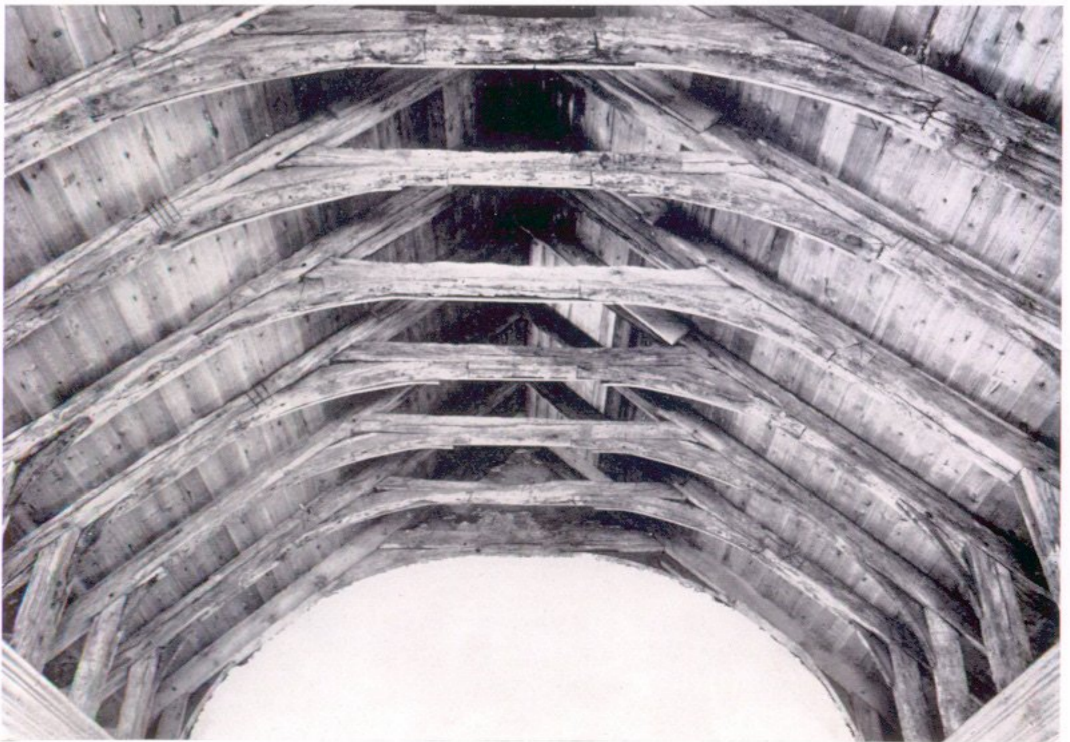
2. The Guthrie Aisle, roof timbers
