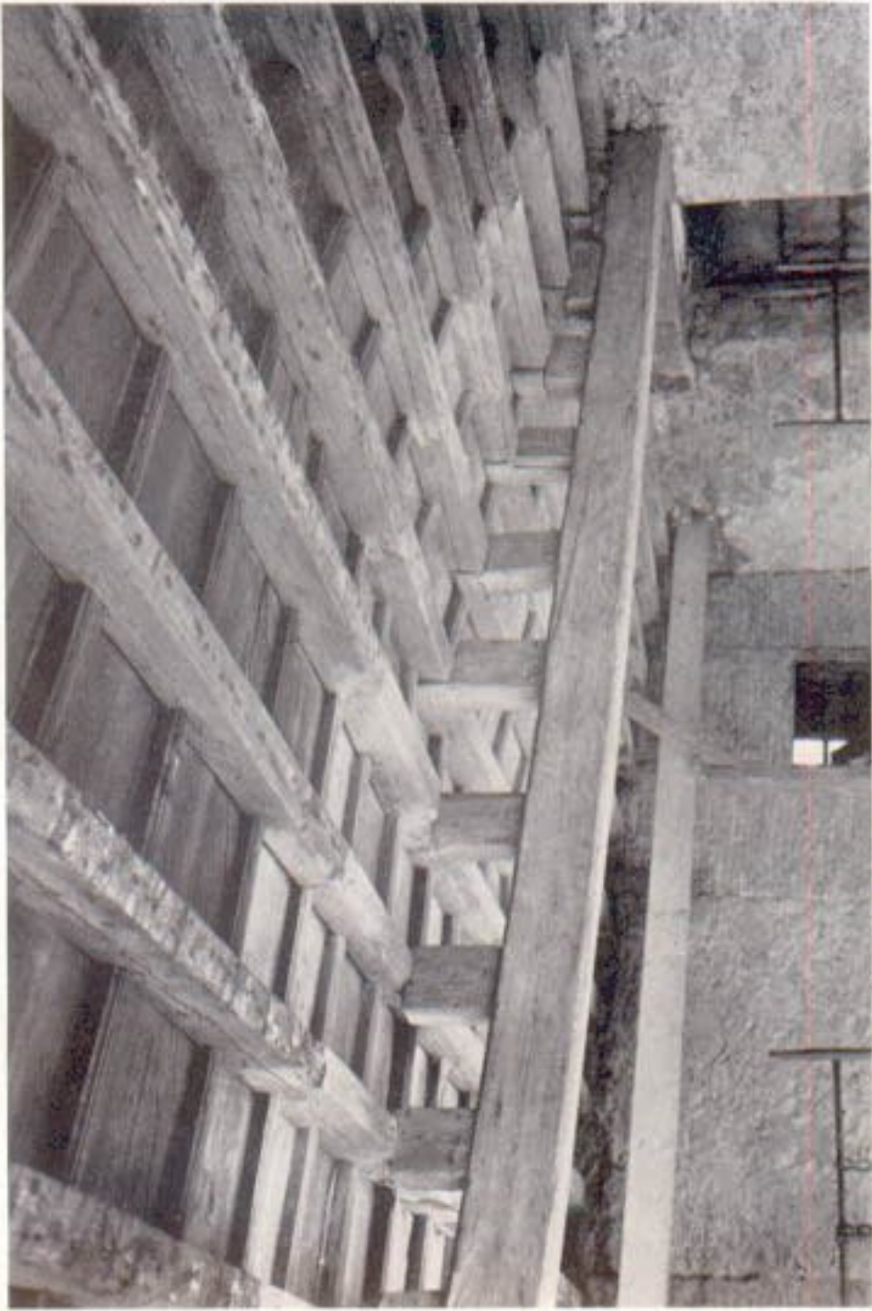
2. West attic chamber: ceiling construction
