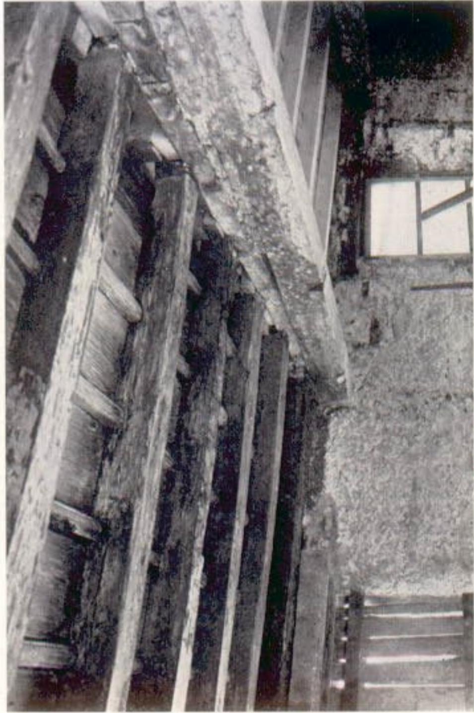
4. Original ceiling of attic: east end
