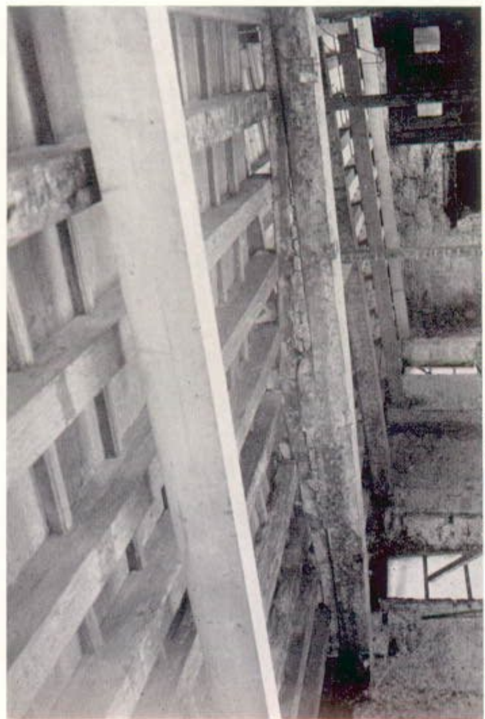
3. East attic chamber: original ceiling
