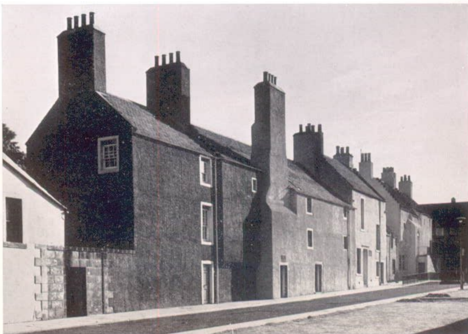
(a) The Watson's east tenement (Mary Somerville's House), north front, after renovation.
