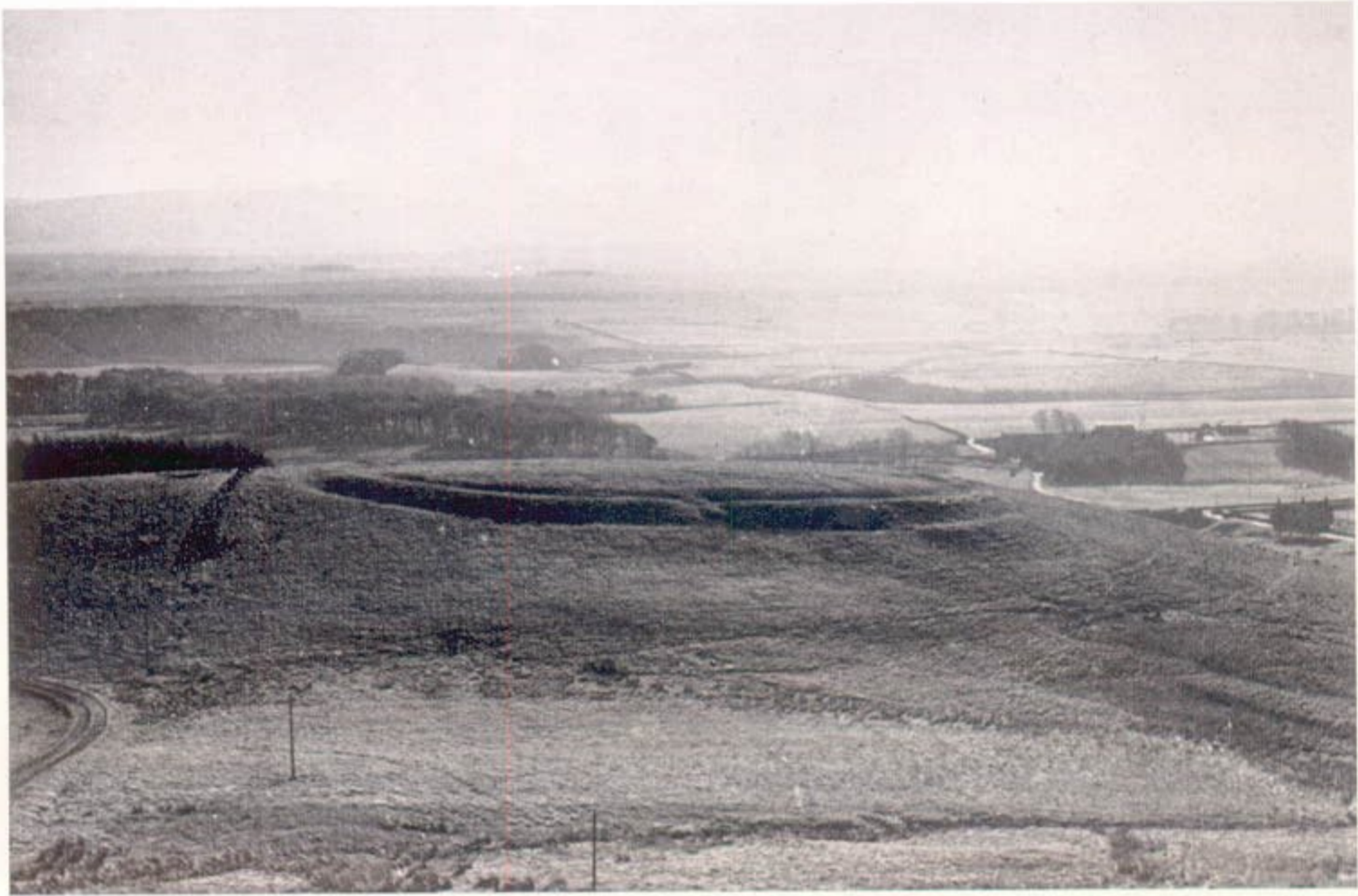
(a) Braidwood Fort from the north.
