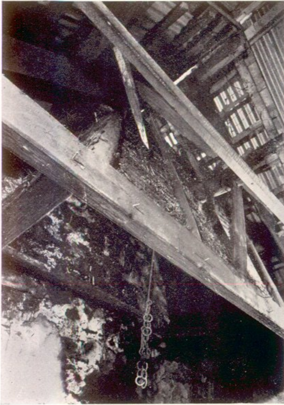
(a) Long House, Camserney, Chimney "B".
