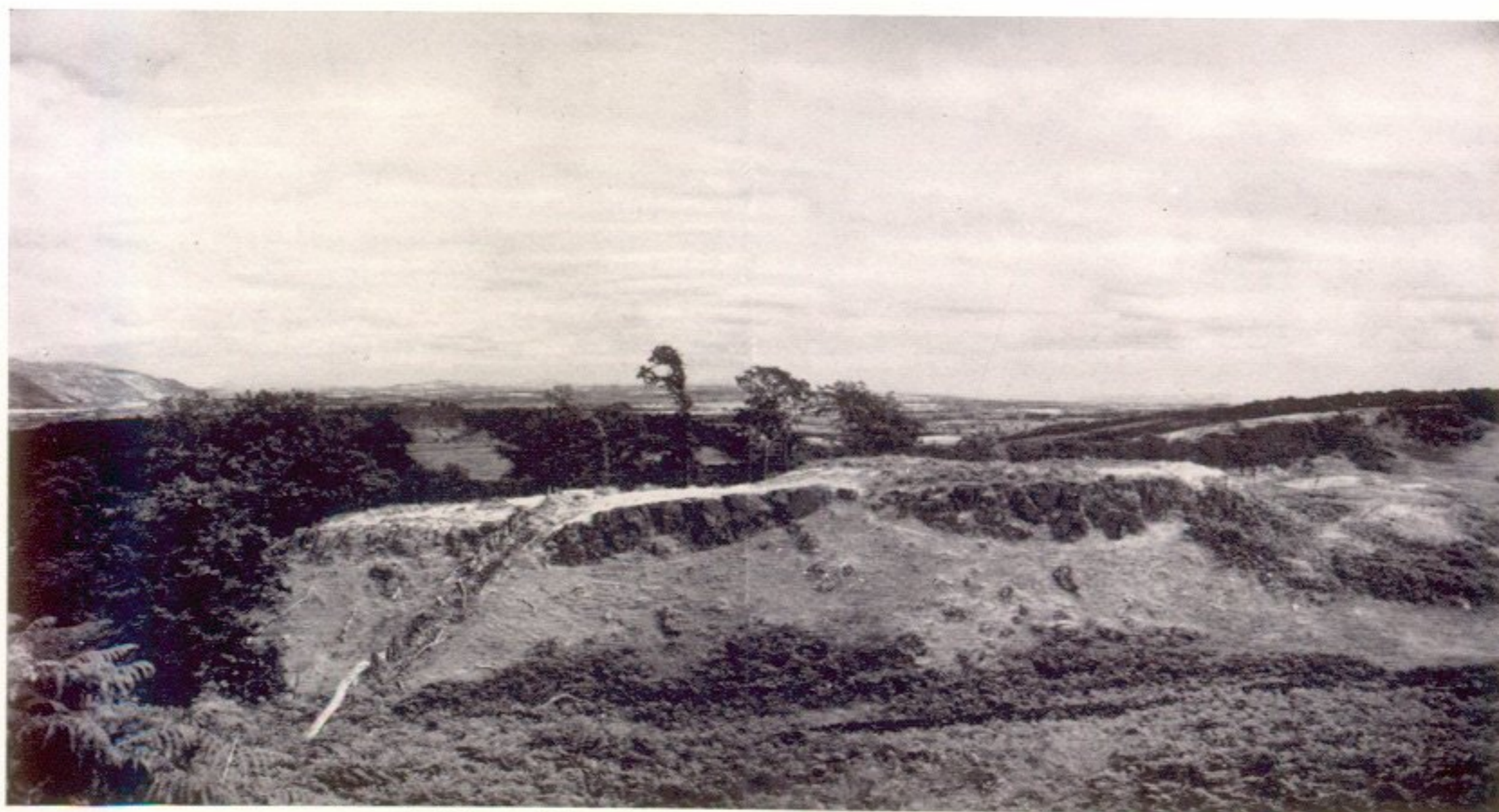
2. View of the site from W. before excavation.
