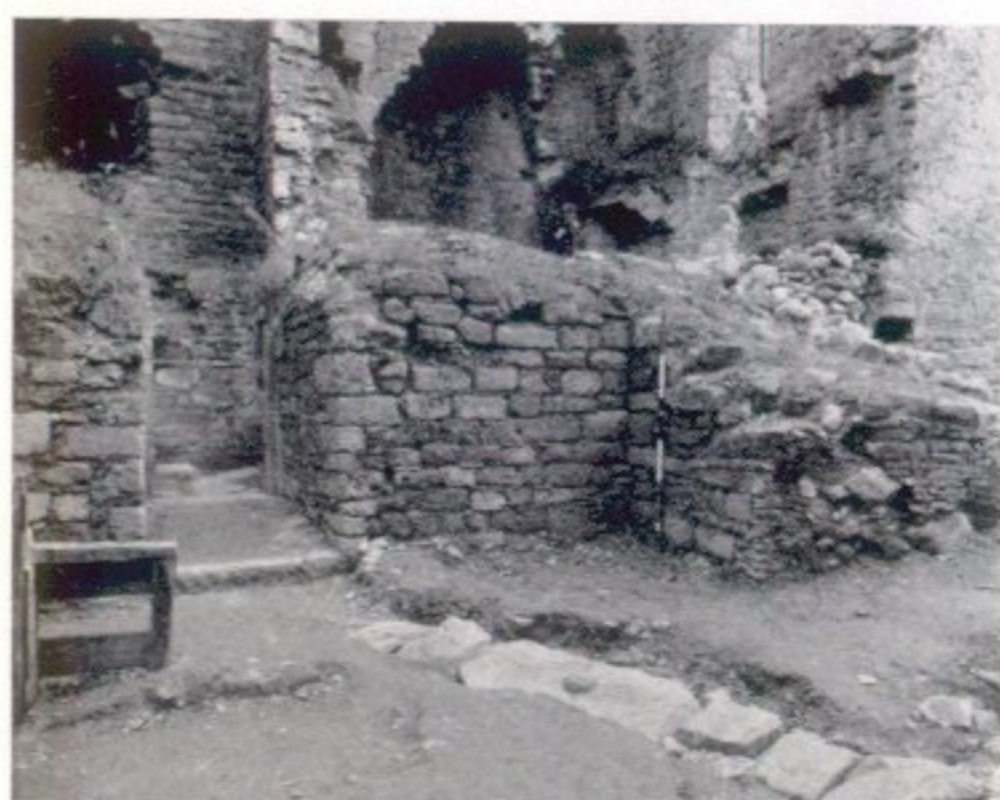
4. Finavon Castle: inner NE. angle of Great Tower. Note floor-drain with bung in situ .
