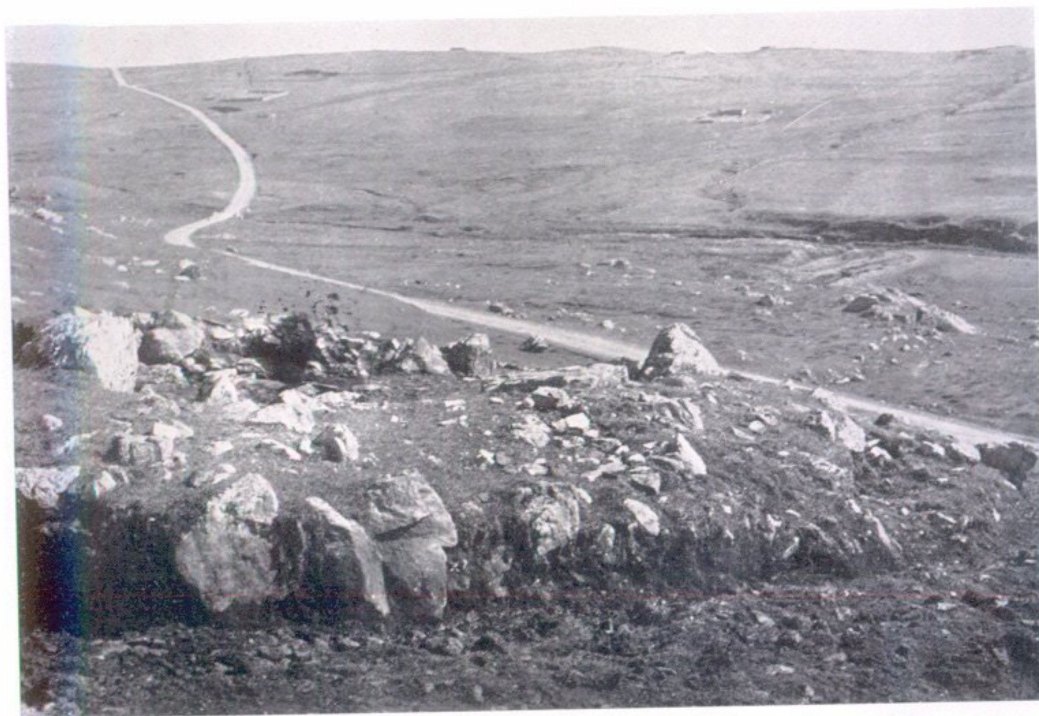
1. View from north-west showing exterior wall-face.
