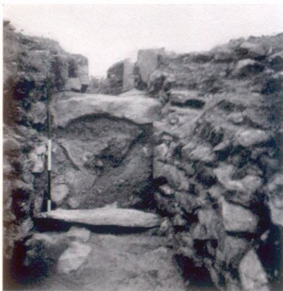
2. Entrance, showing fallen lintel cover.
