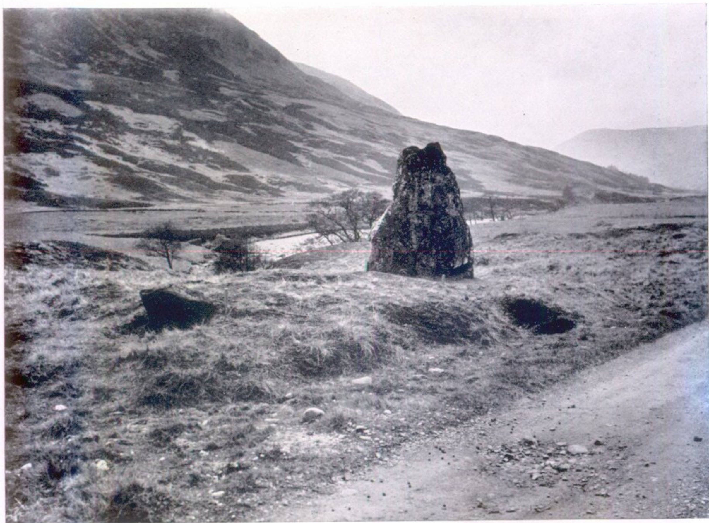
The small cairn from the NE., before excavation.
