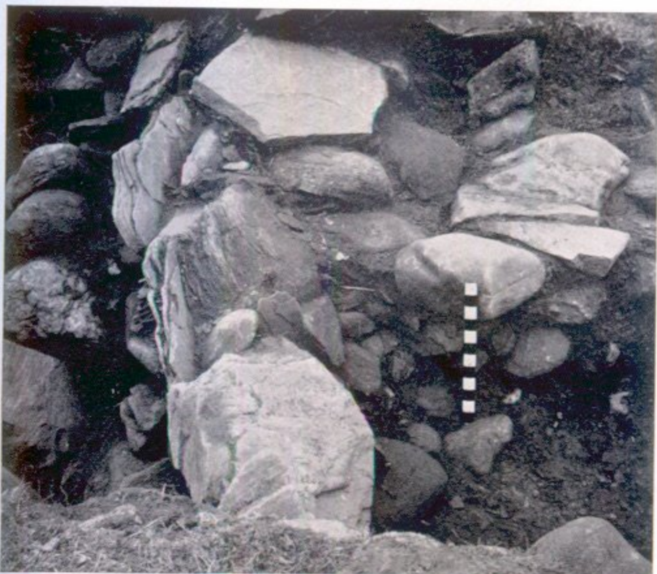
2. Sloping kerb slabs behind Chamber 3 from the east. The cairn material in the near half of the cutting has been removed.
