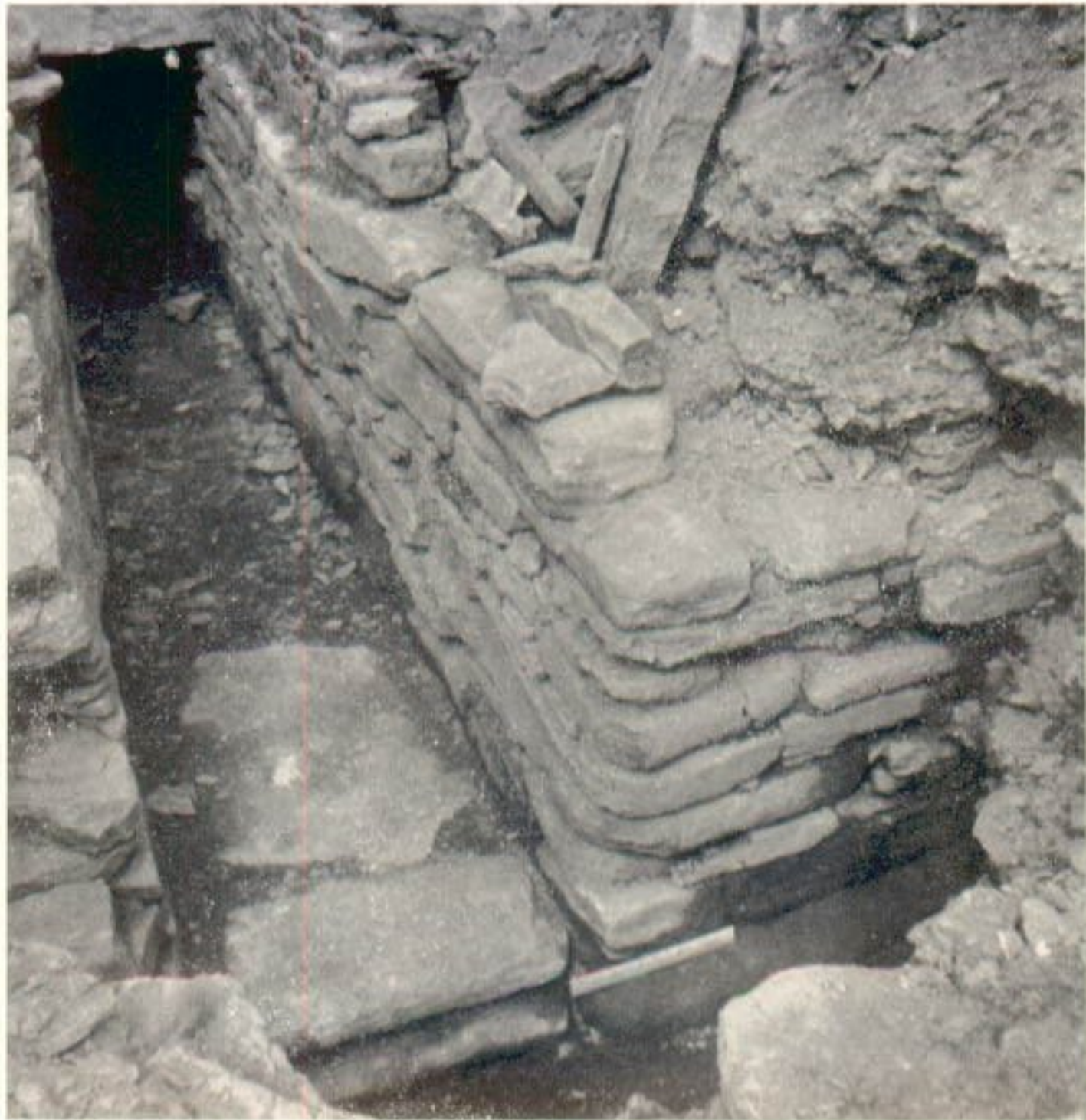
1. Outer end of passage, north side.
