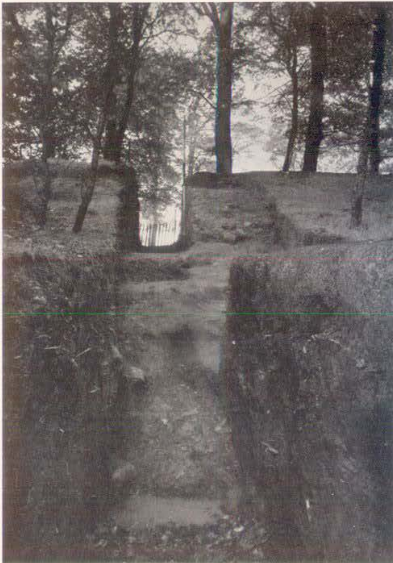
Camphill, Queen's Park, Glasgow: Section across ditch and rampart from outside, near western side of entrance passage.
