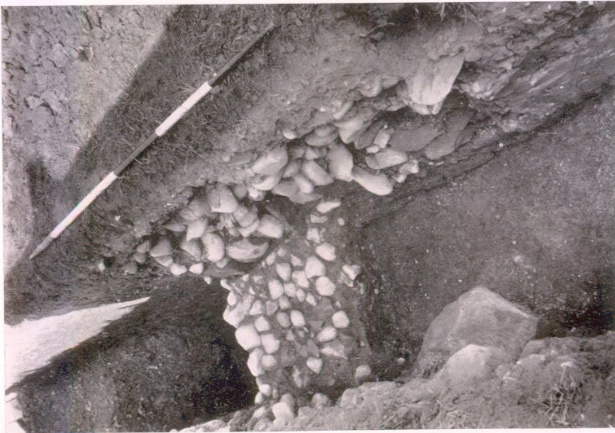
1. Foundation of early Antonine fort-wall (Period III), with cobbled foundation of front of late-Domitianic rampart below and inner Agricolan ditch in background.
