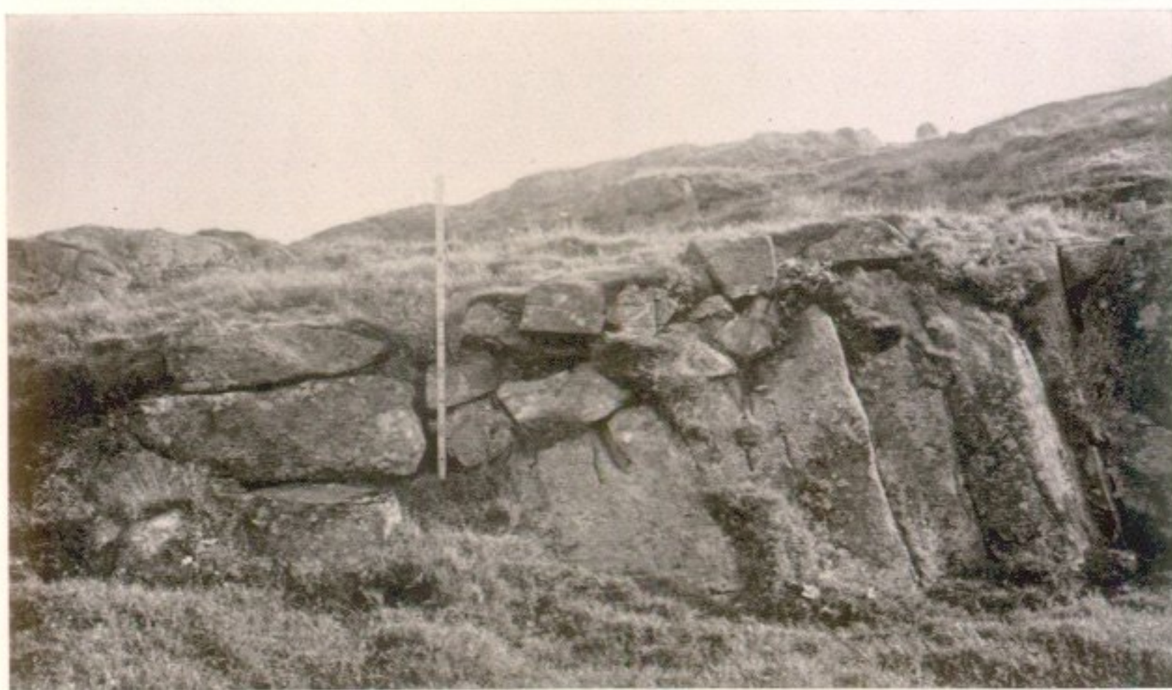
3. Dalmahoy, walling and rock face, north side of enclosure 1.
