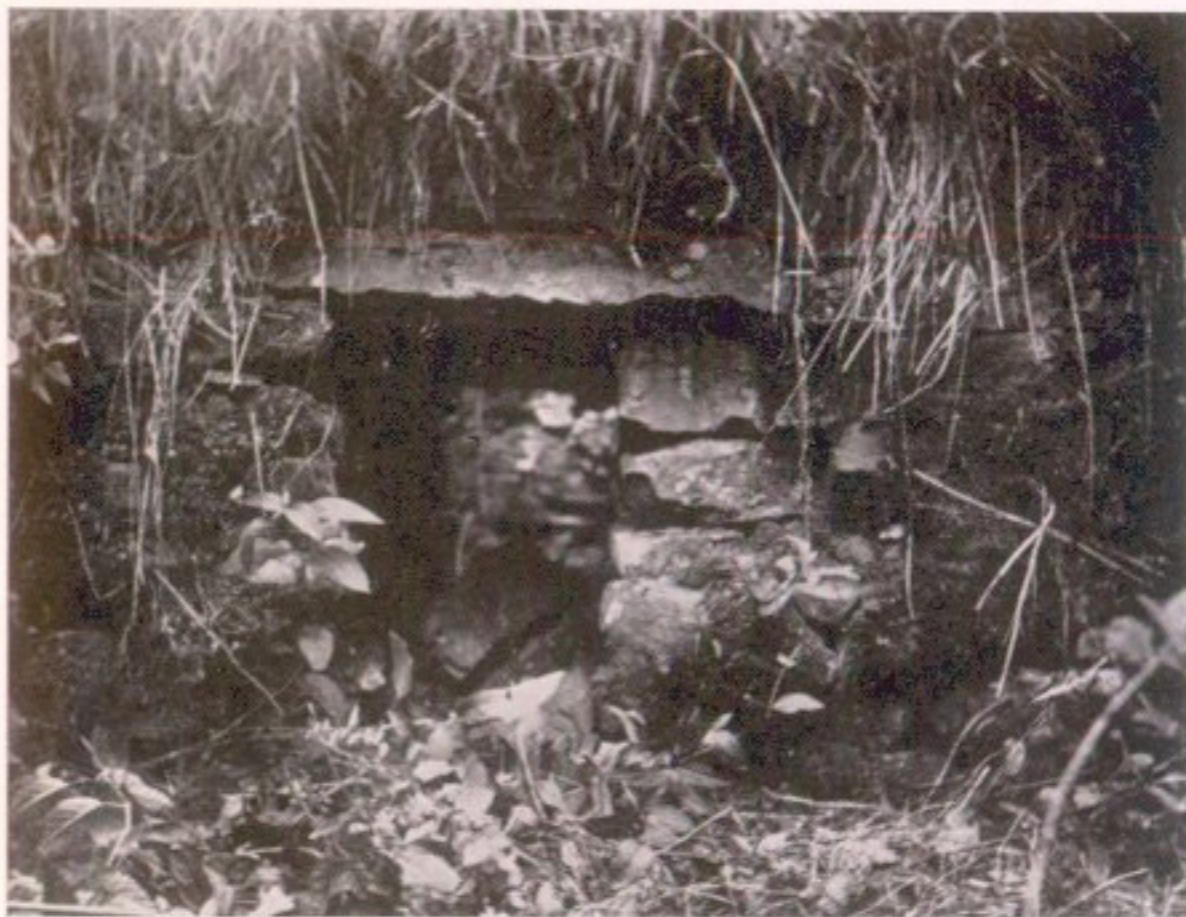
2. Coldoch Broch: entrance to north-western cell.
