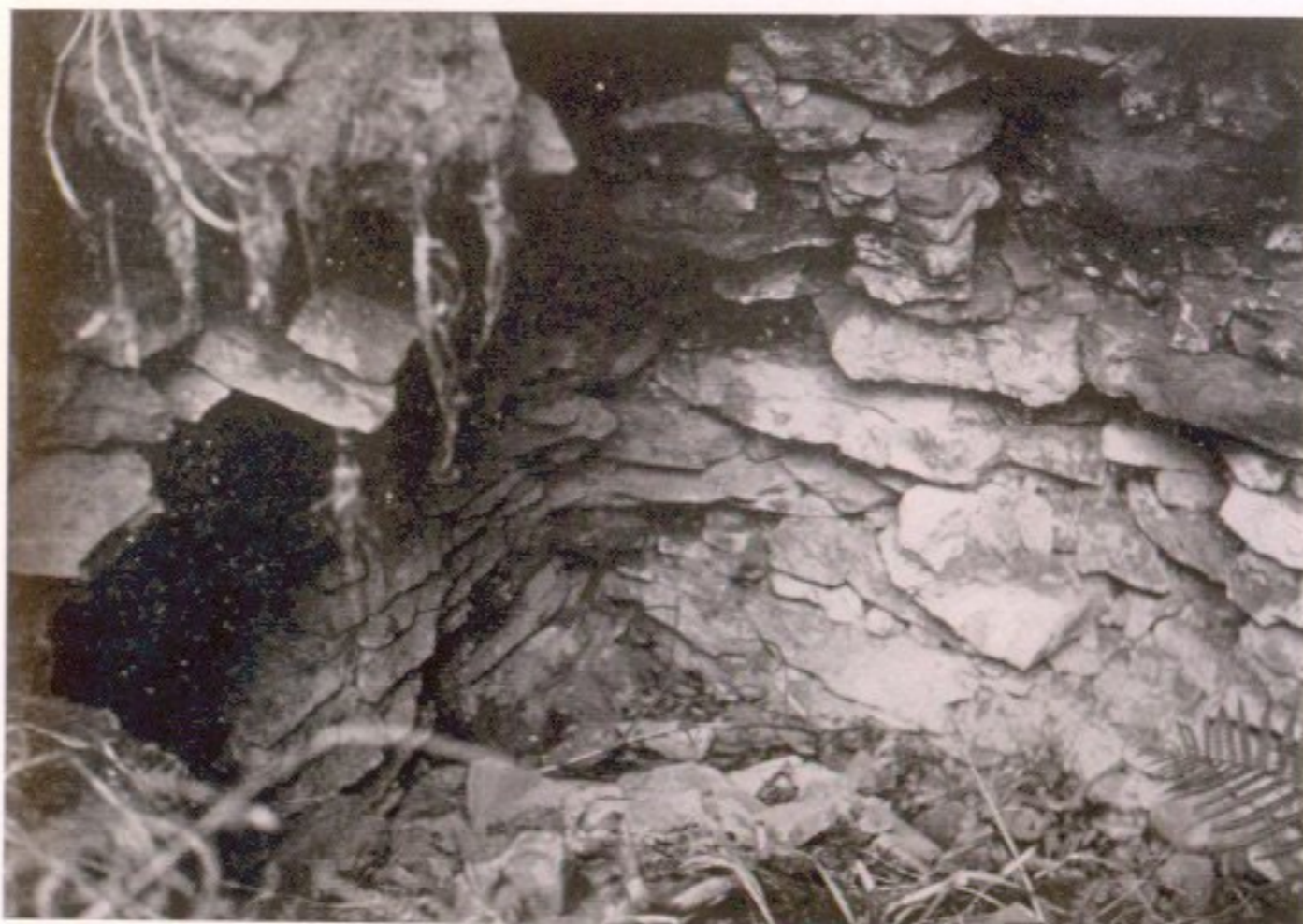
3. Coldoch Broch: interior of northern cell, showing square corner.
