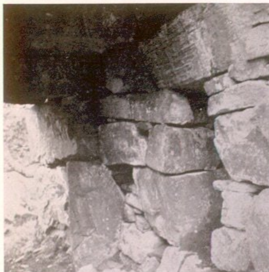
2. Caisteal Grugaig: interior of entrance passage, showing door-check and entrance to guard cell.
