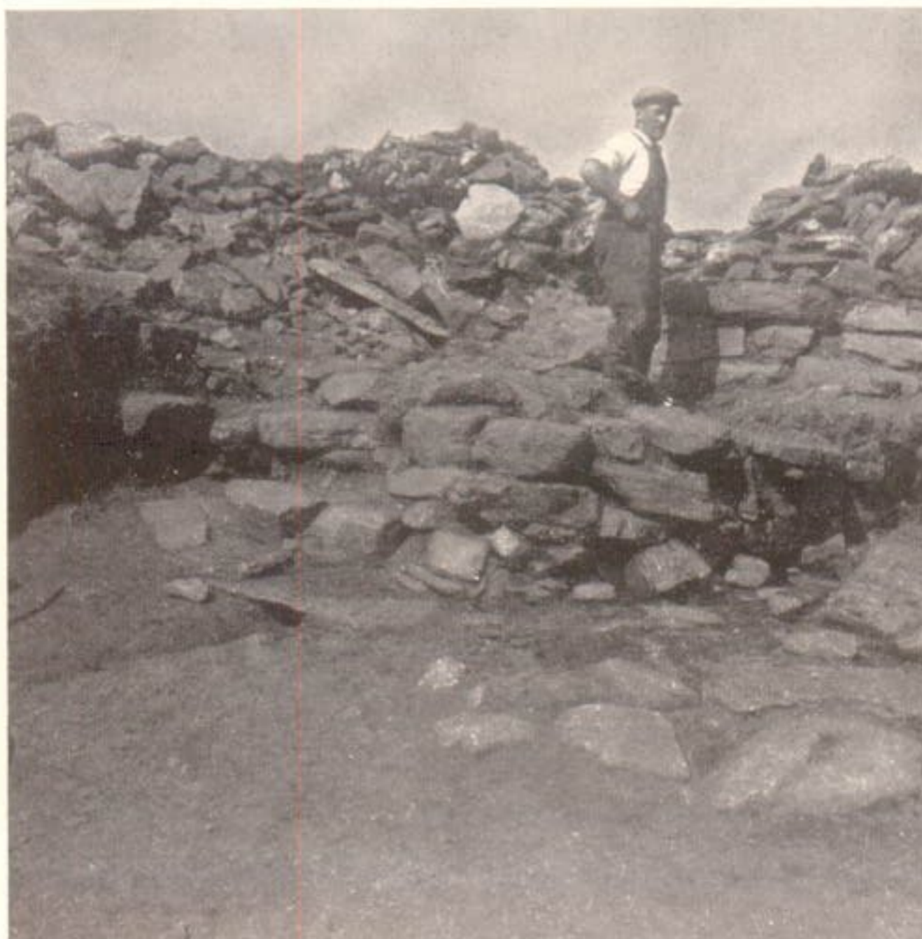
2. South aspect, showing channel passing beneath paving slab subsequently destroyed.
