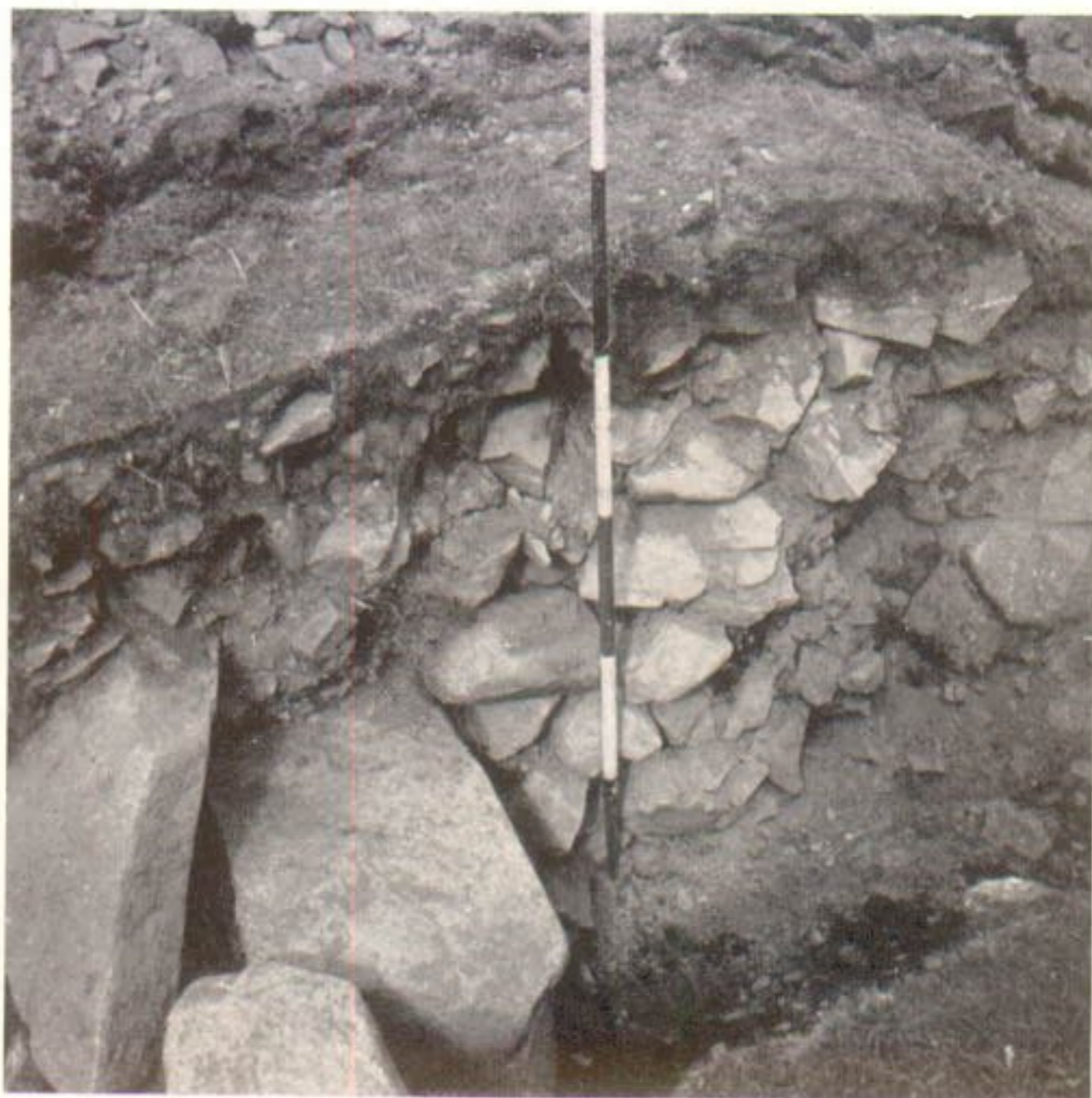
(a) Wall core of Phase II (Area I) with, on left, the facing blocks thrown down in Phase III.
