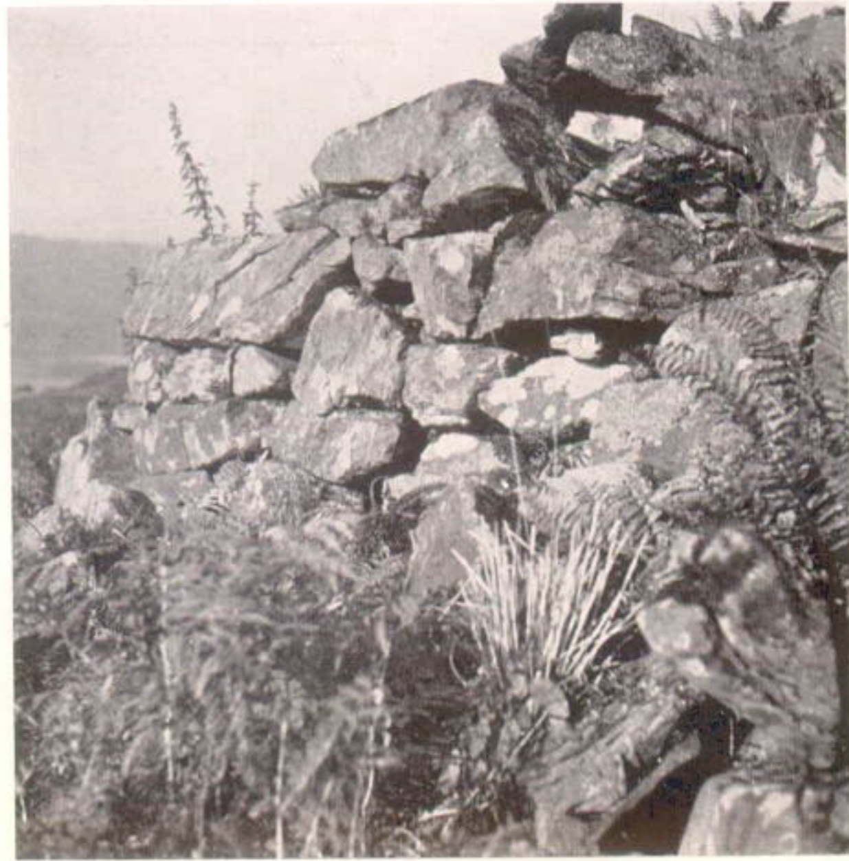
2. Fort below Mullach Dubh; masonry on south-west face.
