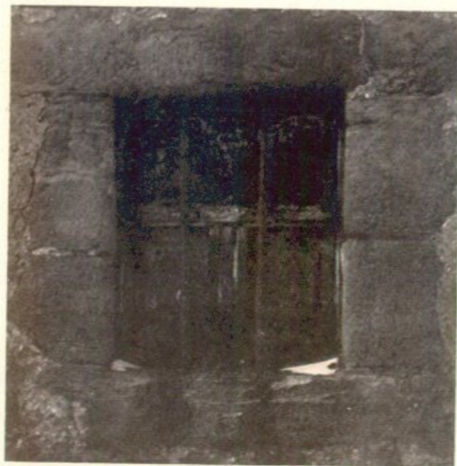
3. Window with panels, at South House, Liberton.
