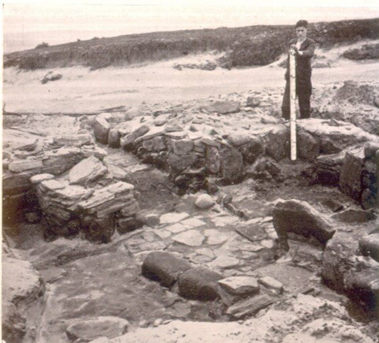
2. West room looking south.
