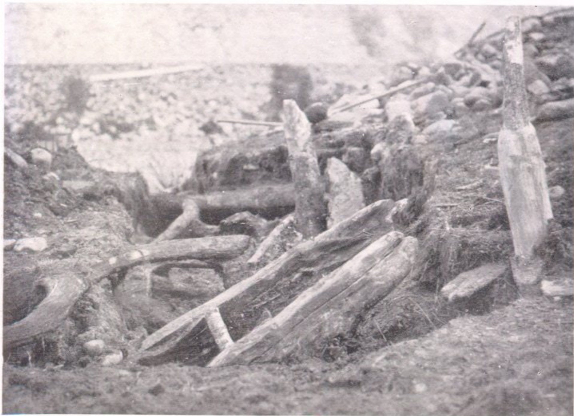
2. Remains of Ladder for access to island.
