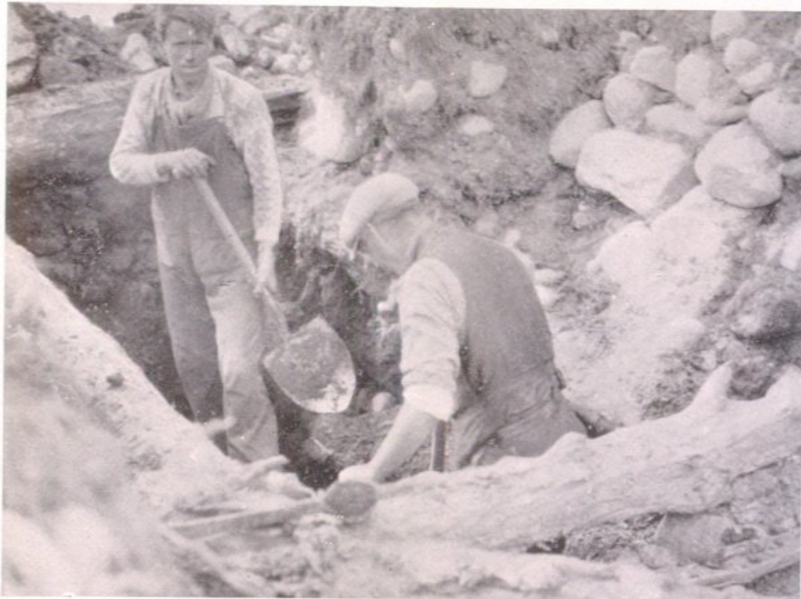
1. Beams of Framework at centre.
