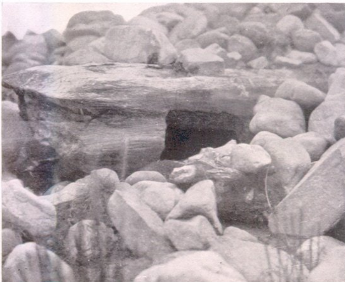
2. End of Cross-beam.
