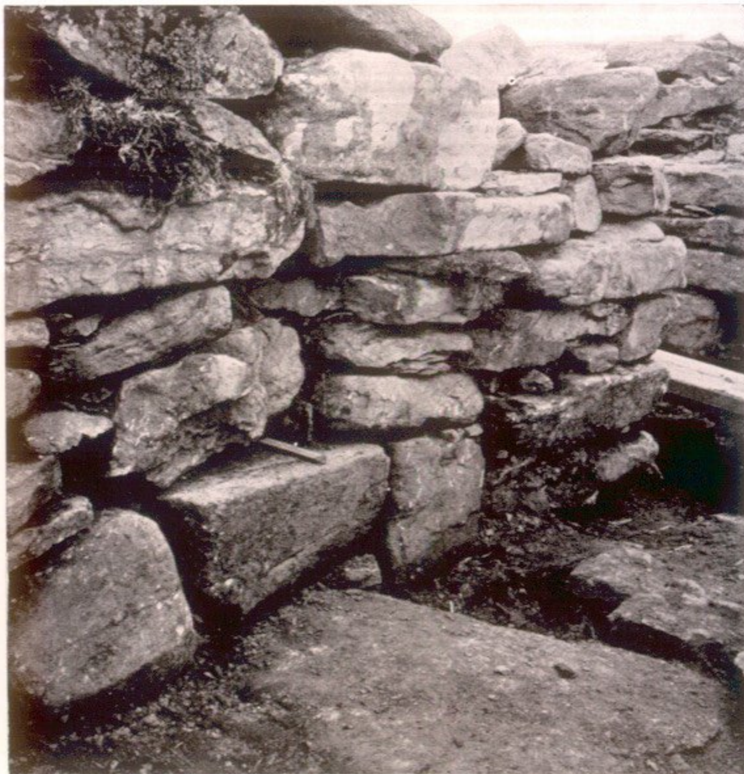
2. South Wall of C: recess at foot-rule.
