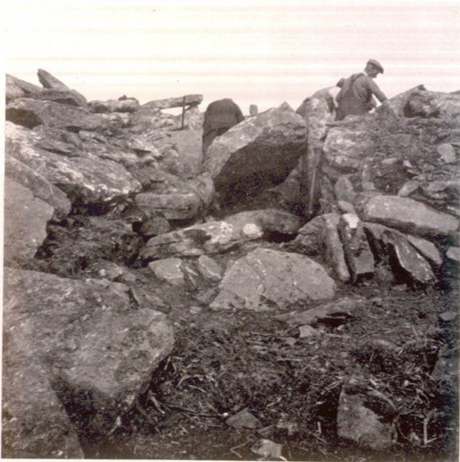
2. Fallen lintel in doorway.
