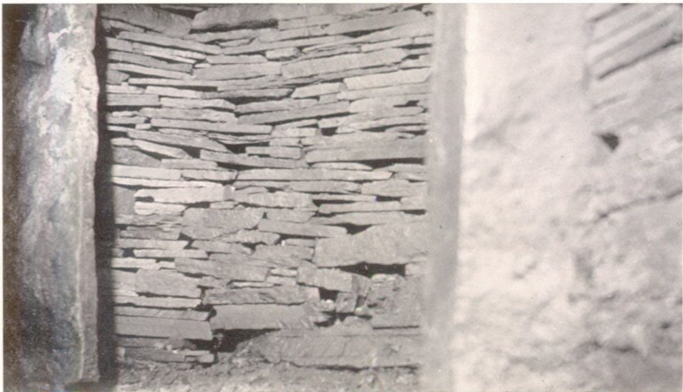
3. Detail of Masonry. The Miniature Chamber.
