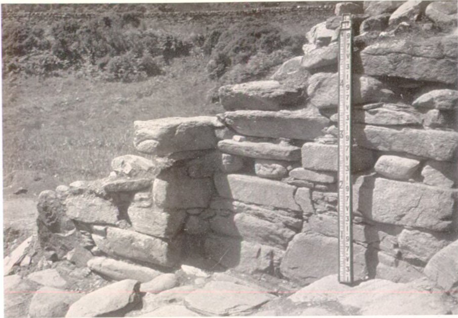
1. The north wall of the Entrance, Period I.
