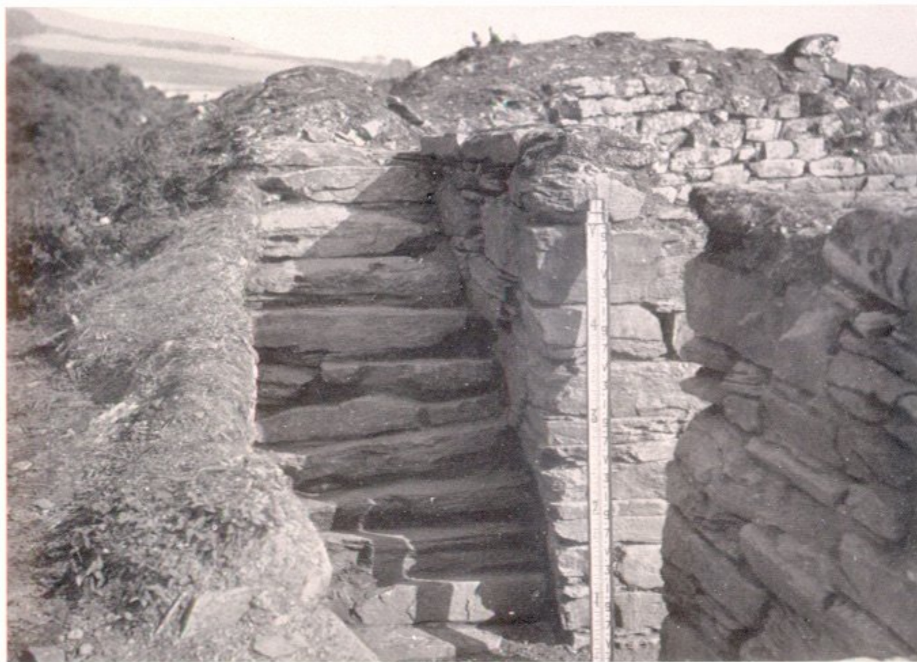
2. The north Stairs, with the Staircase Entrance on the right.
