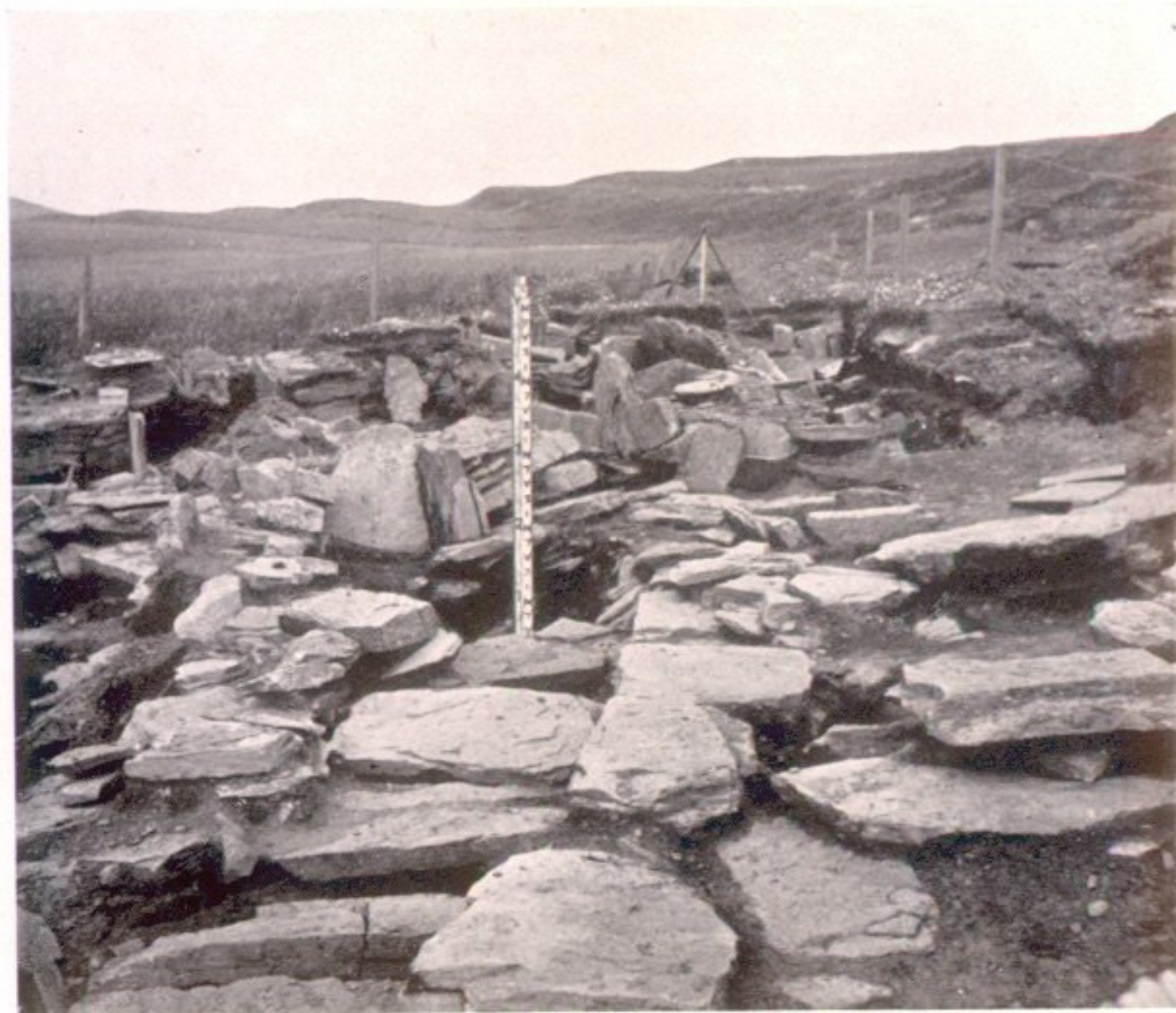
2. Drain under Chamber B, looking north.
