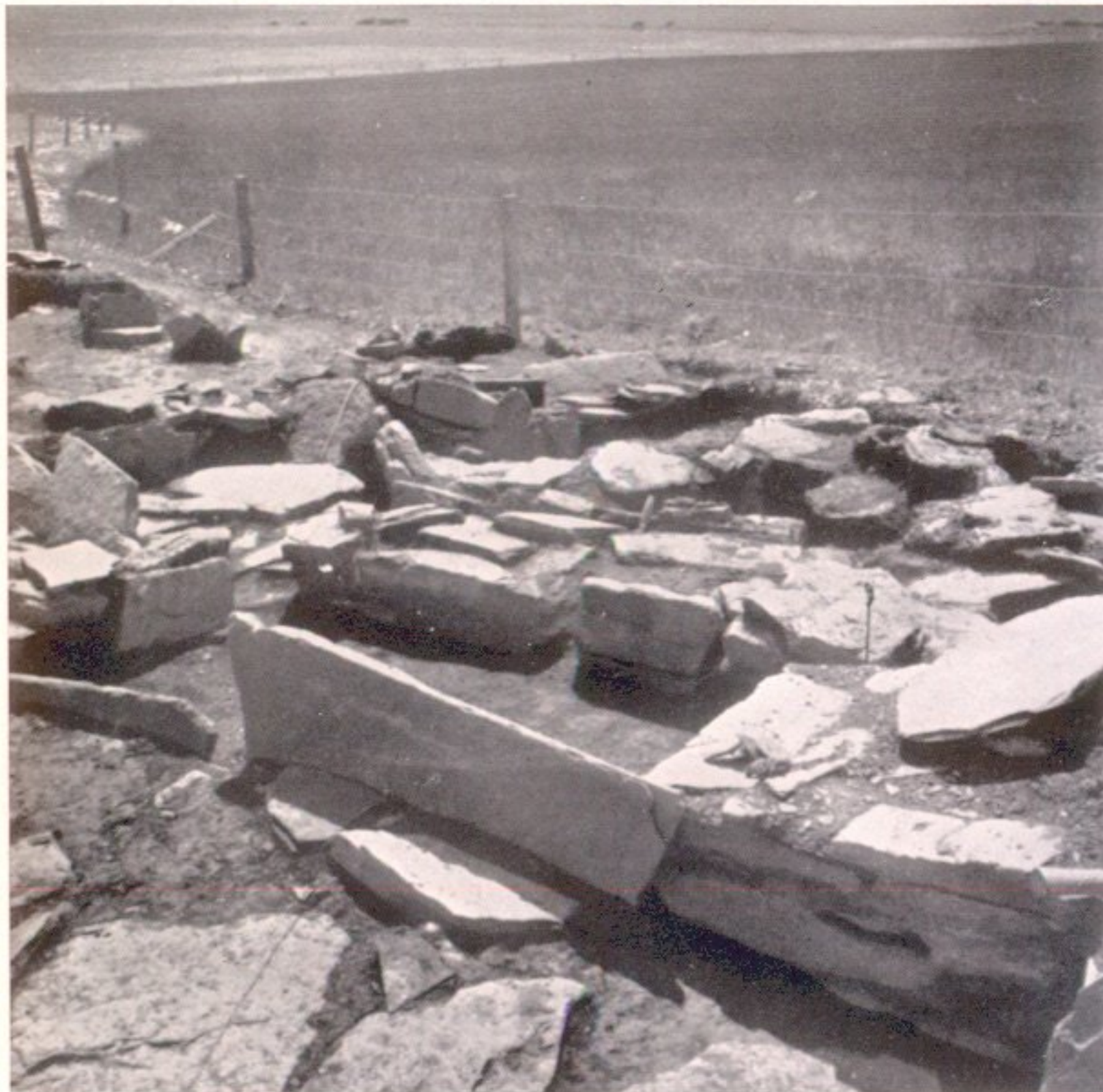
1. Right-hand bed of Chamber A, looking south.
