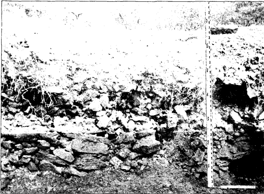
Fig. 4. Inner Face in north-west Quadrant and Culvert (right).
