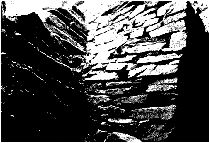
Fig. 4. Torr's Cave: Platform-Structure and Stairway.
