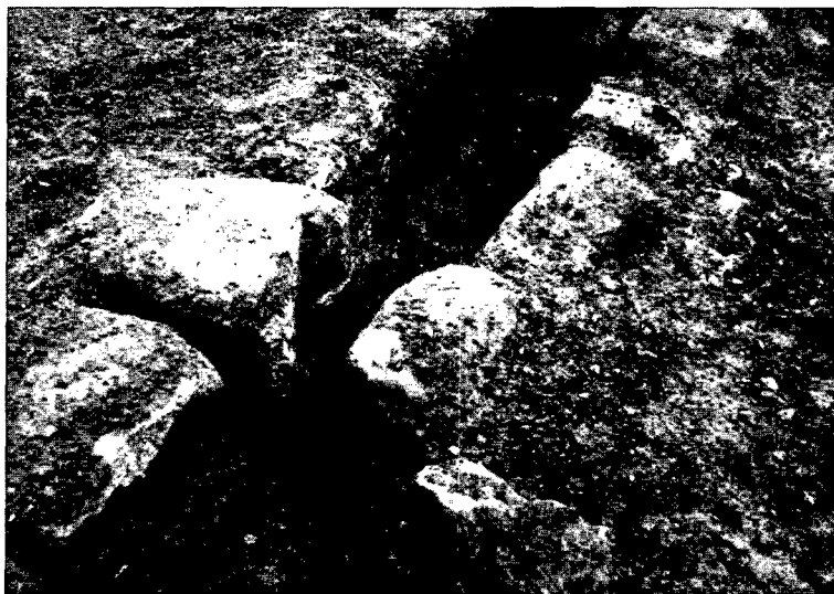
Fig. 9. Built channel underneath the floor of the Ambulatory, showing constriction. The stone in the foreground is displaced.
