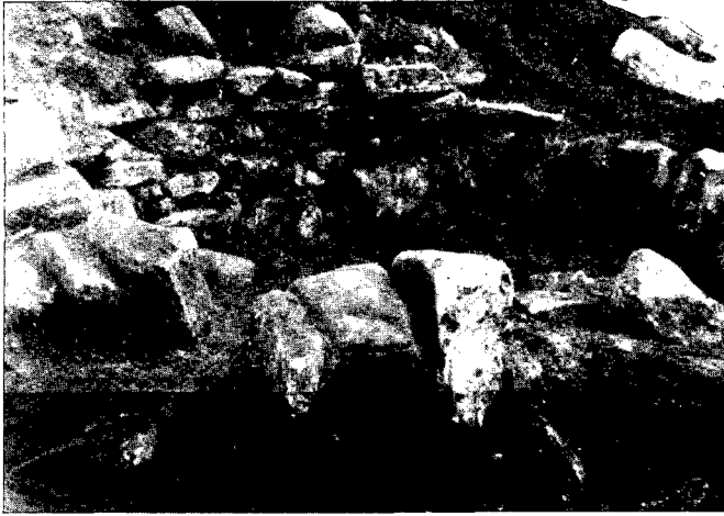
Fig. 2. Secondary Hut abutting on Wall of Fort east of Entrance.
