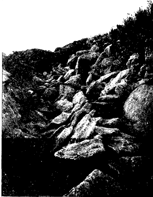
Fig. 11. Peristalith looking west from Q. 6. The inner wall of large blocks is on the right, the intermediate wall of flat slabs is to the left of this, and the outer ramp of tilted slabs is further to the left.
