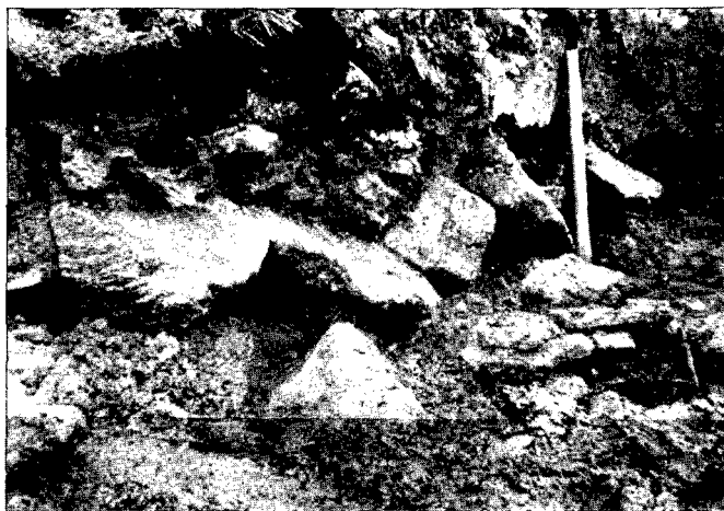
Fig. 10. Abutments of northern Façade. Section of dry walling in front of Pick.
