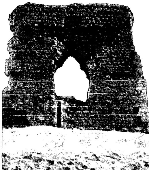
Fig. 4. Dunnideer Castle: view of tower from west.
