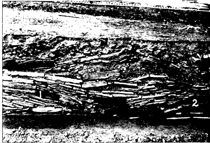
Fig. 5. Midhowe Chambered Cairn, showing face of Outer Wall with String Course and slant of stones reversed (1) and (2).
