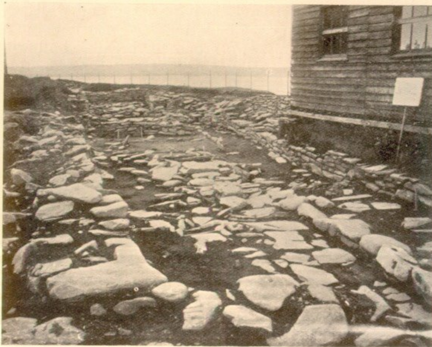
Fig. 2. The Interior from the South End after excavation.
