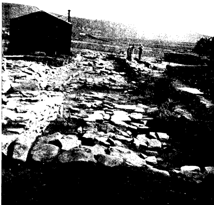
Fig. 4. The Interior from the North End.
