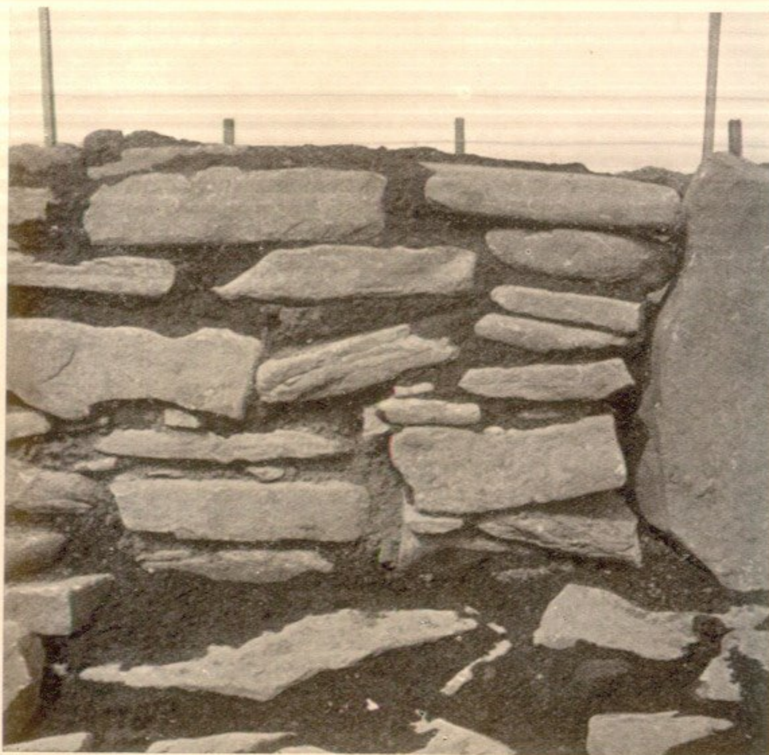
Fig. 3. Inner face of Wall showing Method of Construction.
