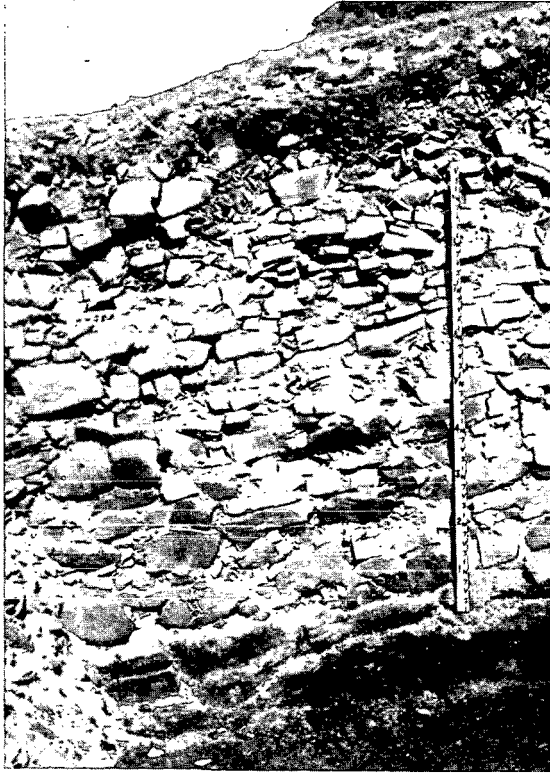
Fig. 10. Inner face of wall in Section D (the staff is truly vertical).
