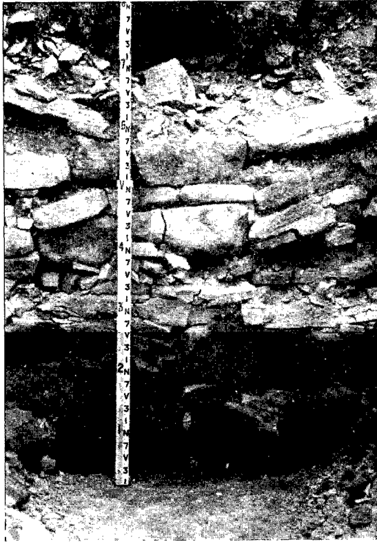
Fig. 6. Outer face, north rampart.
