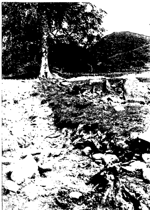
Fig. 3. The Northern Kerb, looking east.
