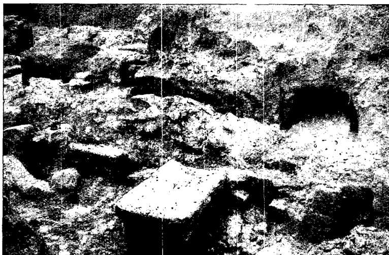
Fig. 45. Portion of south wall of Men's Baths, showing (a) in the foreground the remains of partition wall dividing Caldarium from Tepidarium, (b) to the right of it two of the recesses for heat flues, and (c) behind these one of the buttresses.
