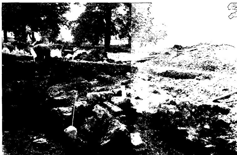
Fig. 46. Opening up the stoke-hole of the Caldarium in Men's Baths. The fallen mass to right of the yard measure represents the remains of three brick pillars that had flanked the entrance.
