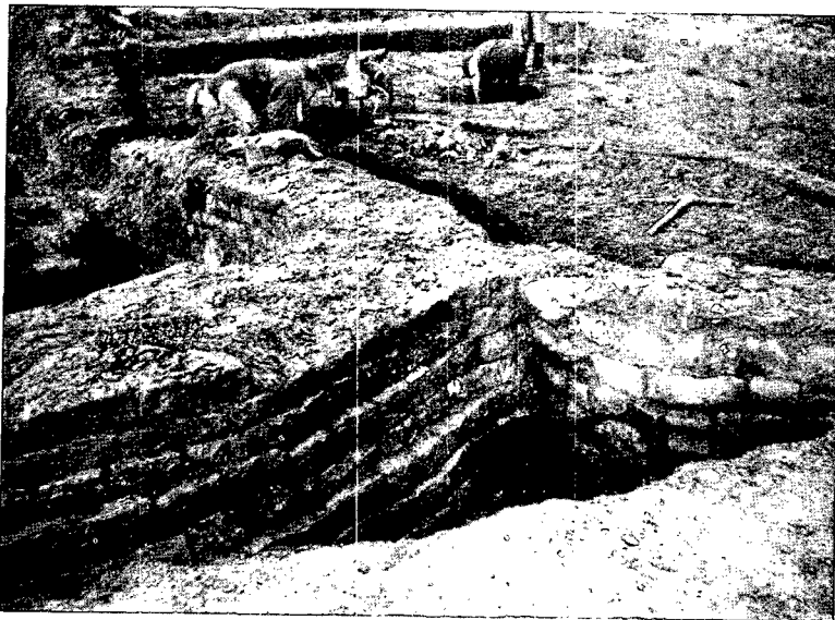
Fig. 60. Outer face of the apse containing the cold bath, with remains of paving of the Apodyterium in the background.
