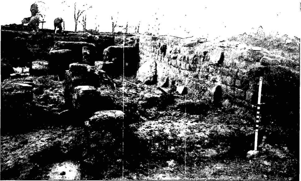
Fig. 53. Caldarium of Large Bath-house, looking west. The view is taken from the furnace-room, where the three levels were most clearly marked.
