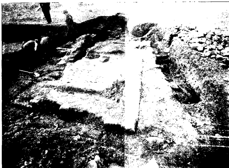
Fig. 44. General view of Apodyterium of Men's Baths, looking west. The stokehole of the Sudatorium is just being opened up.
