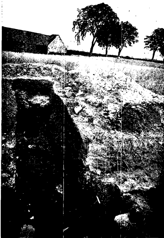
Fig. 74. Main drain passing out of the fort underneath Antonine Wall, the level of the kerbing of which is indicated by the top of the spade. The blocking of clay and stones can be seen towards the farther or north end.
