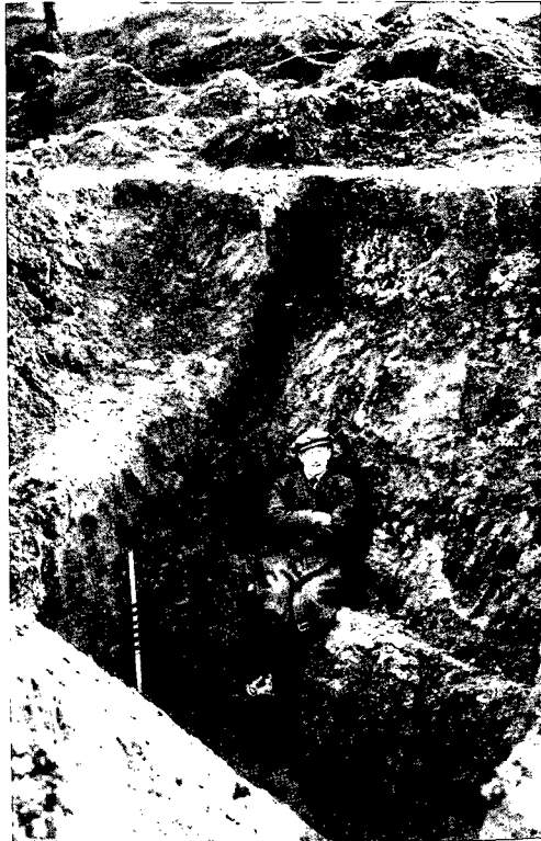
Fig. 13. Counterscarp of innermost ditch on the west, showing well-defined ledge.
