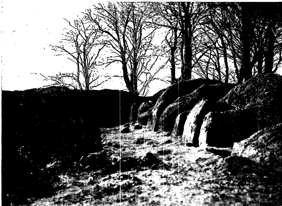
Fig. 28. Remains of foundations of West Granary.
