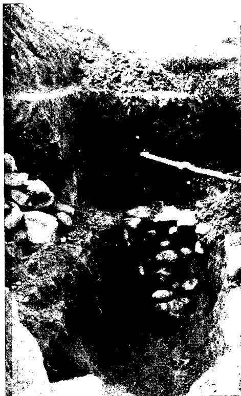
Fig. 10. Pit for foundation of south pier of archway at west gate, partially cleared.
