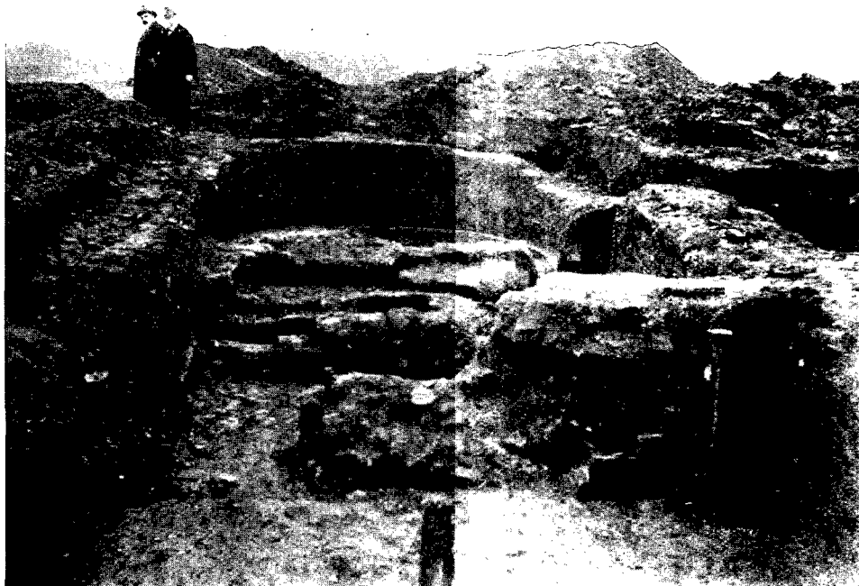
Fig. 58. Frigidarium of Large Bath-house, as seen from Caldarium (C). The drain for the cold douche appears in the middle distance, and beyond are the remains of the low seat in front of the cold bath. For the channel in the middle foreground see p. 482.
