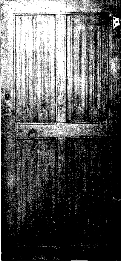
Fig. 8. Door at St Salvator's College, St Andrews.
