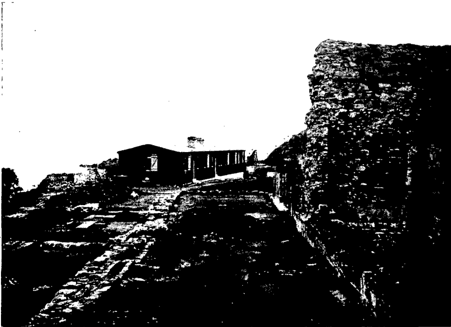
Fig. 3. Inchcolm Abbey: Foundations of Church showing Mural Chamber in North Wall.
