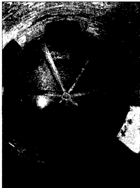
Fig. 6. Vaulted Ceilings, N.W. Tower.
