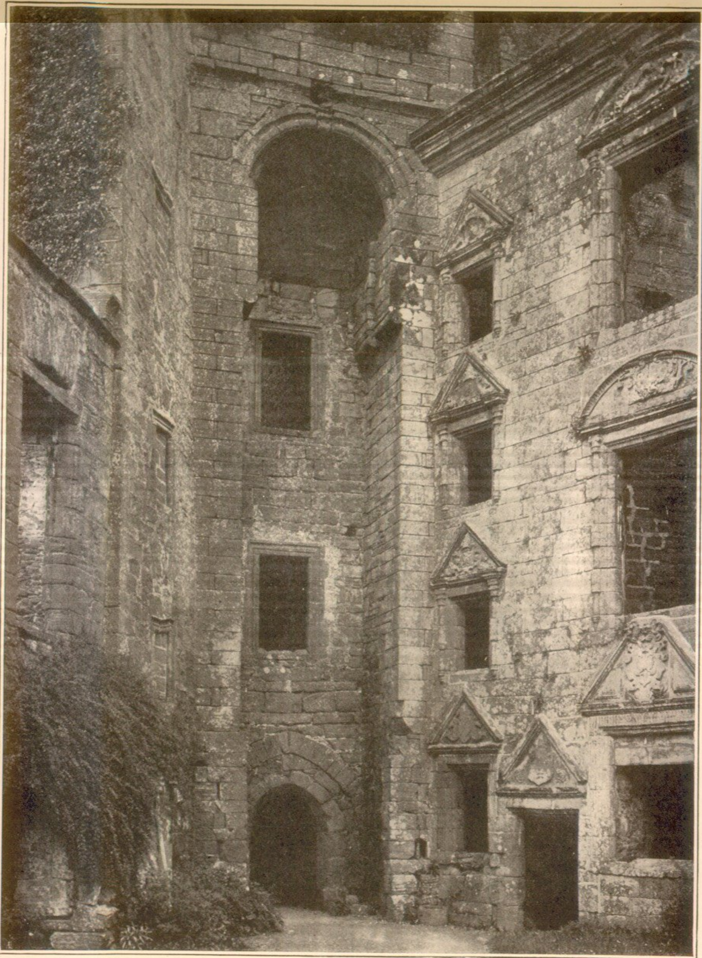
Fig. 8. Caerlaverock Castle : North angle of Courtyard.
