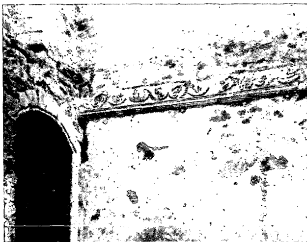
Fig. 3. Huntly Castle: Plaster Work on partition wall.
