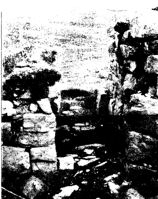
Fig. 3. Entrance, from the interior.
