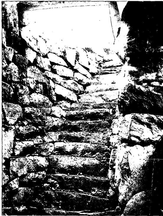
Fig. 5. Remains of Stair.
