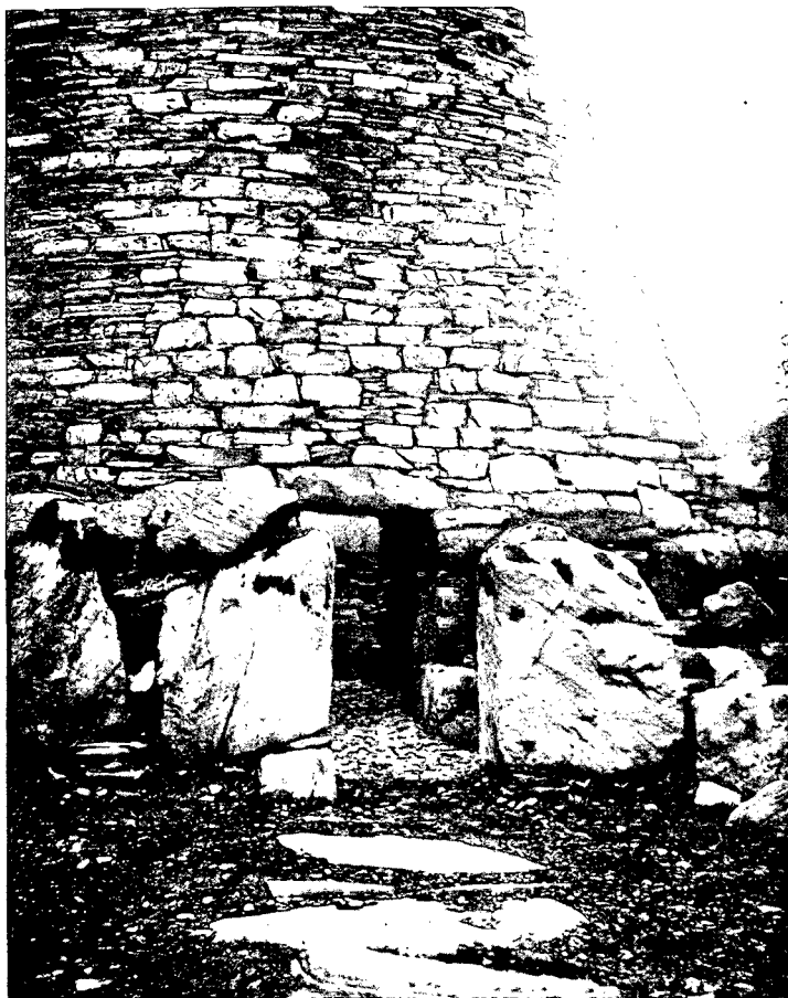
Fig. 8. Dun Telve—view towards the Entrance from outside.
