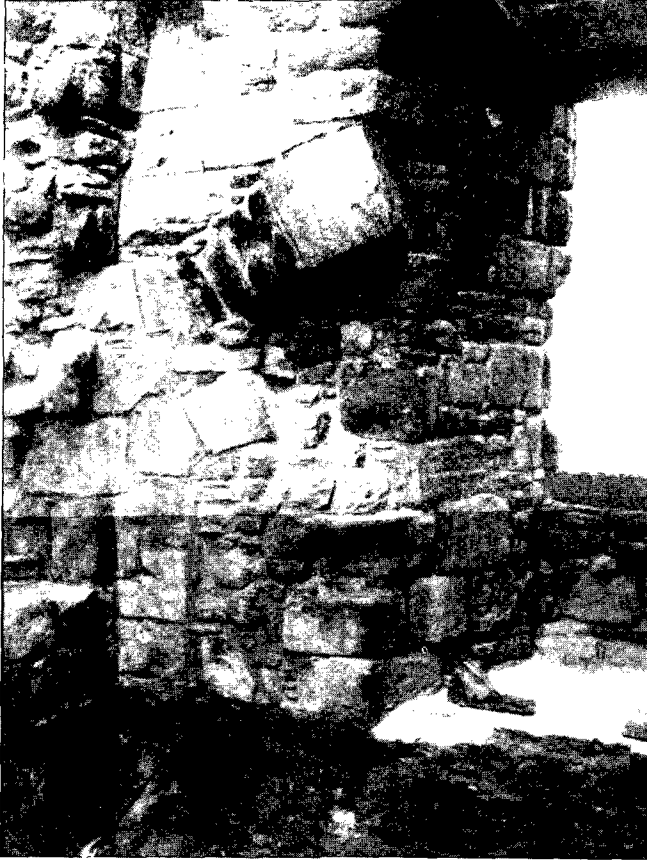
Fig. 11. Interior of Fore Tower of St Andrews Castle.
