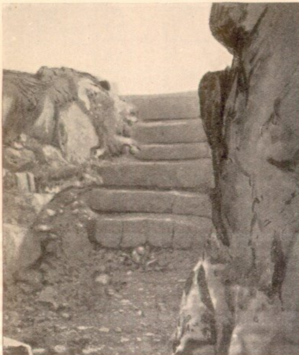
Fig. 5. Remains of the Stair.
