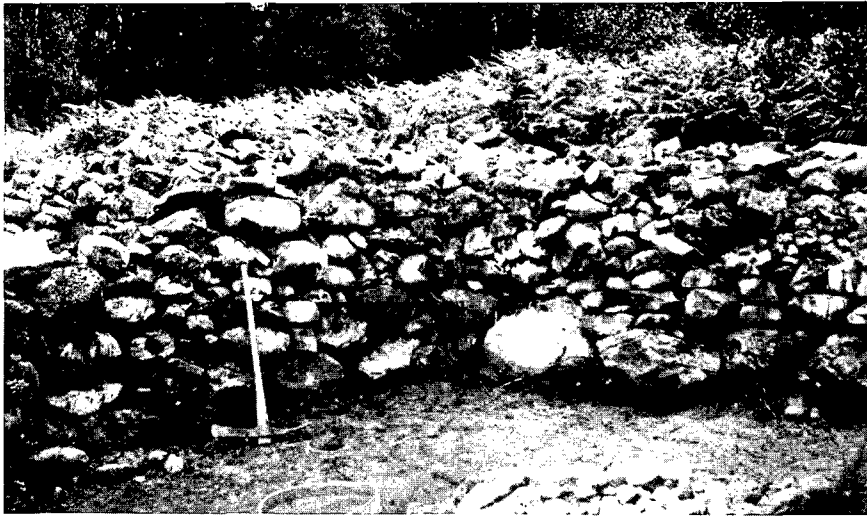
Fig. 11. Masonry of the Inside Wall of the Fort.
