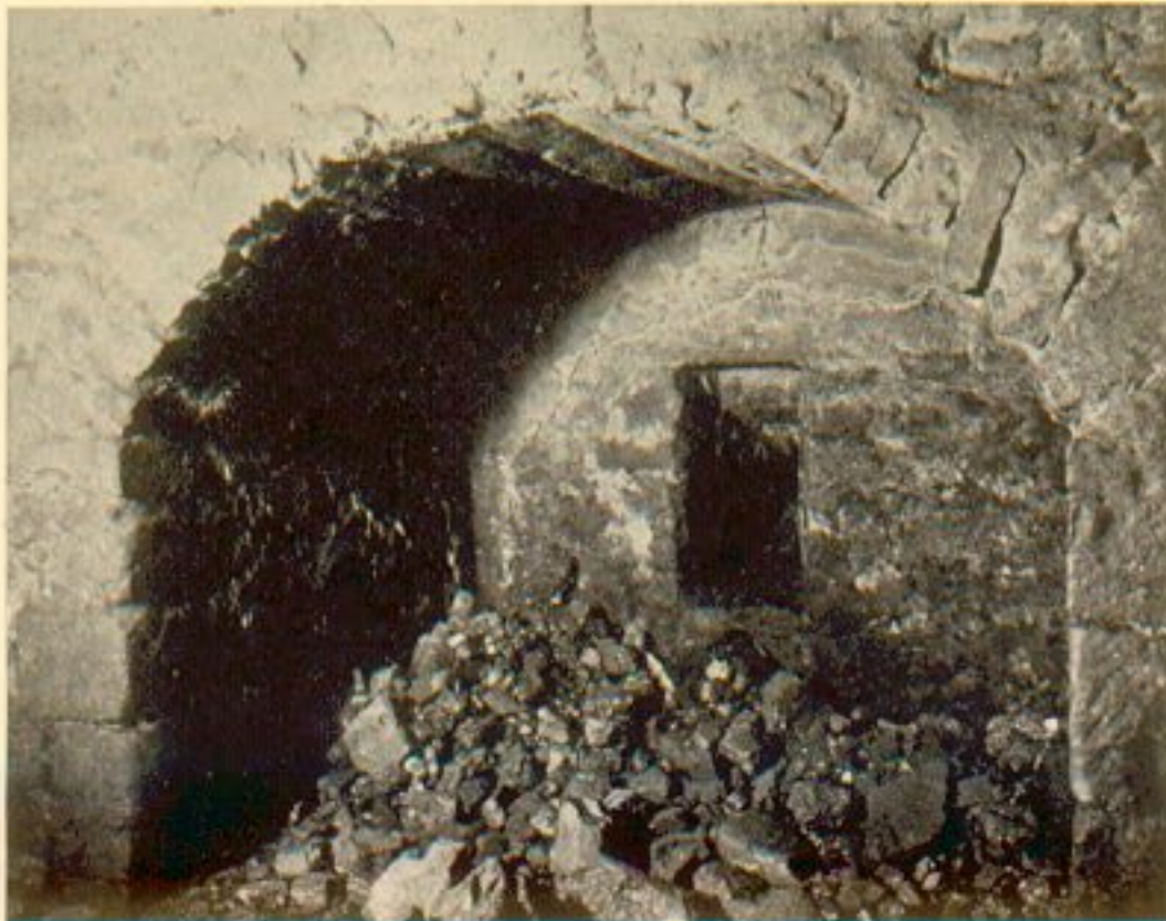
Fig. 5. Canteen Coal-cellar until 1912.
