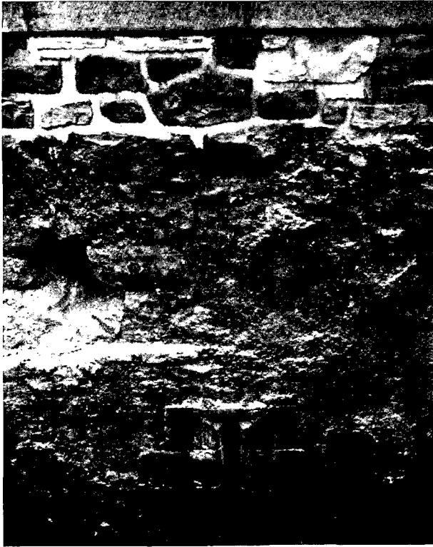
Fig. 7. Outer face of Original Wall of Tower where first exposed.
