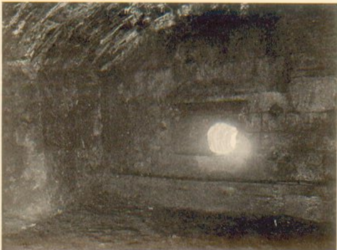
Fig. 16. Vaulted Recess of Battery with Shot-hole.
