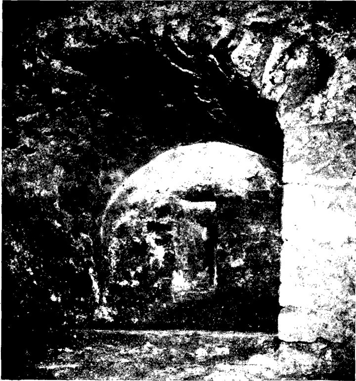
Fig. 6. Vaulted Recess with Shot-hole (after removal of coal-cellar floor).
