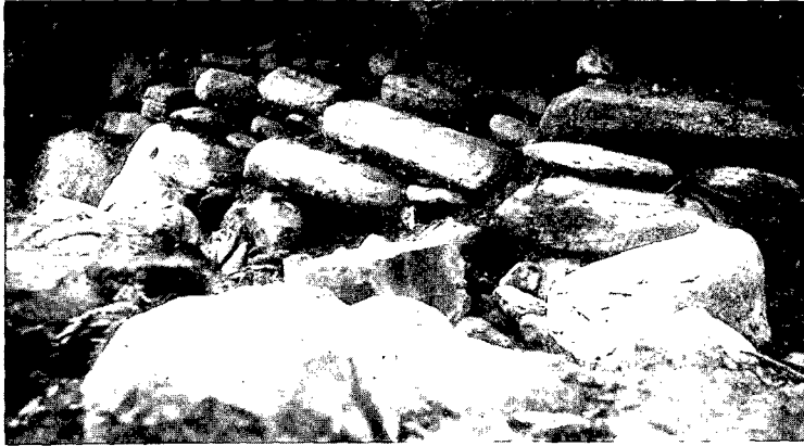
Fig. 6. Part of the Retaining Wall.
